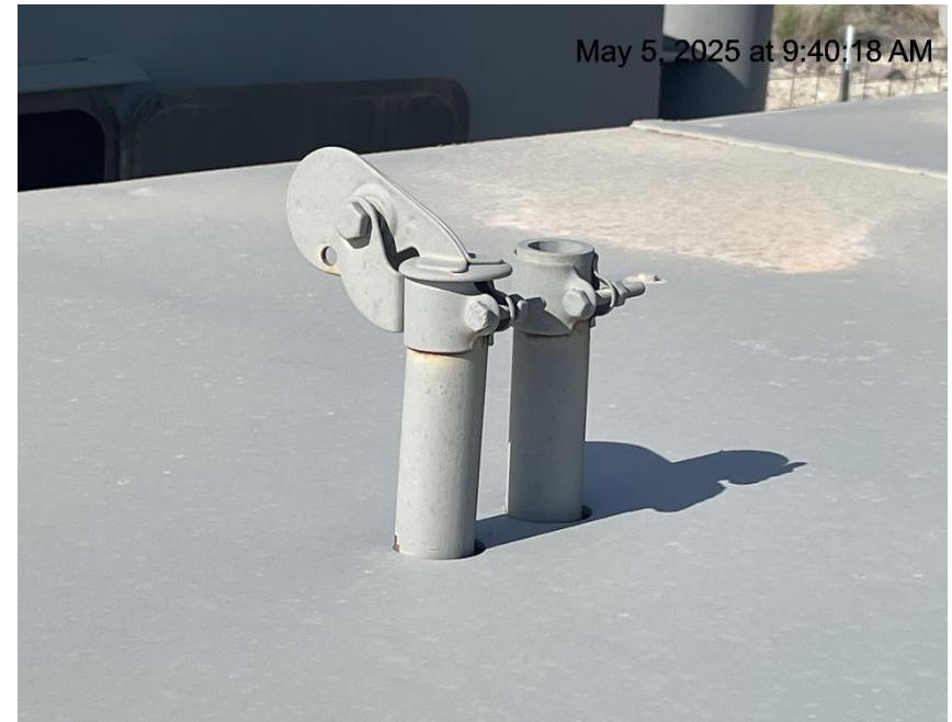
Photo # 8656 PRV vent line does not comply with CECMC pressure safety device rules
