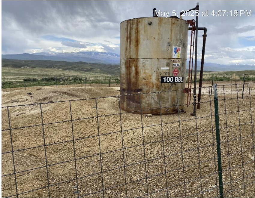
Tank berm insufficient
