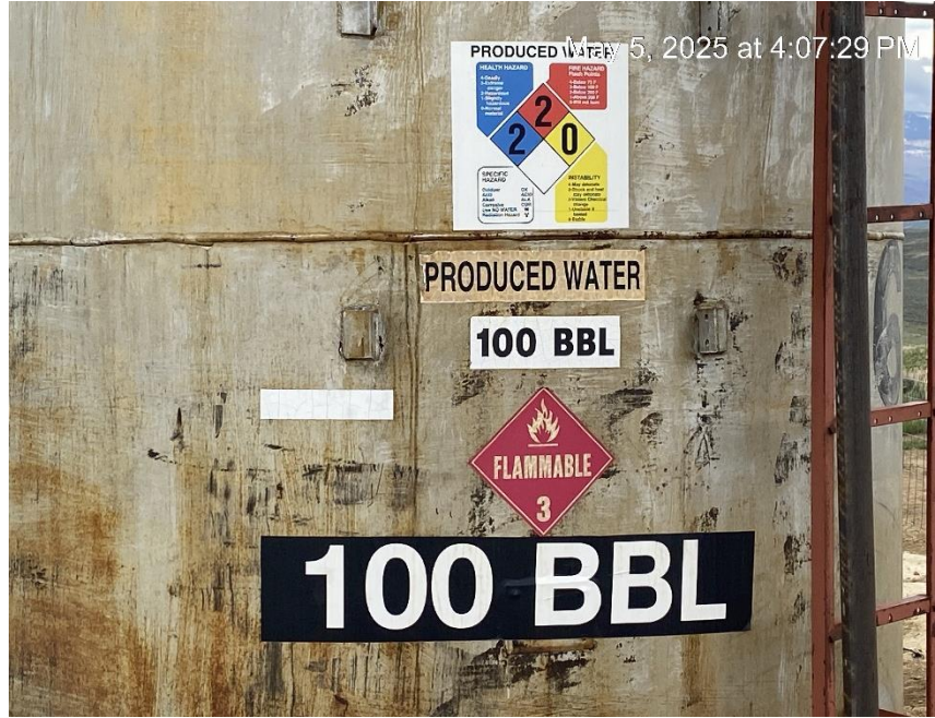
Missing required information
