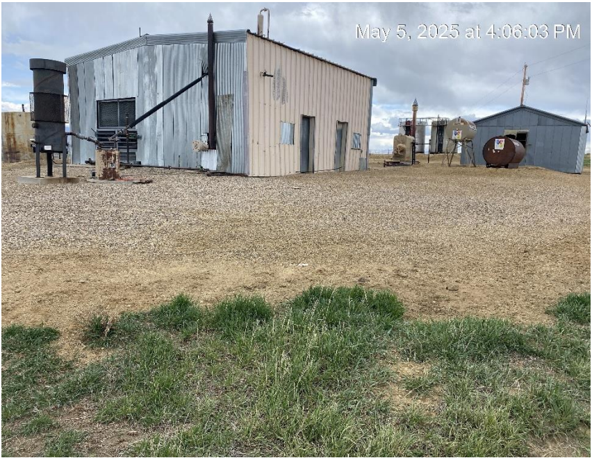
Location from Southwest corner
