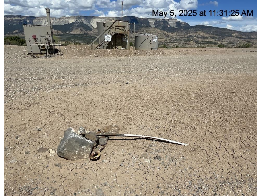
Photo # 8912 Same improperly marked deadman
