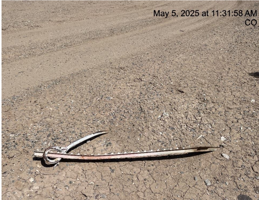
Photo # 8913 Improperly marked deadman
