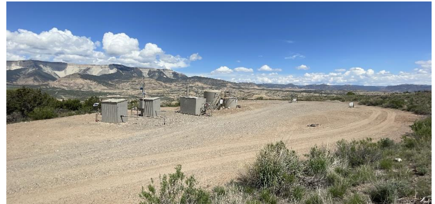
South East corner of location.
