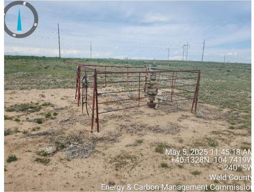
Photo 2 well head and equipment
