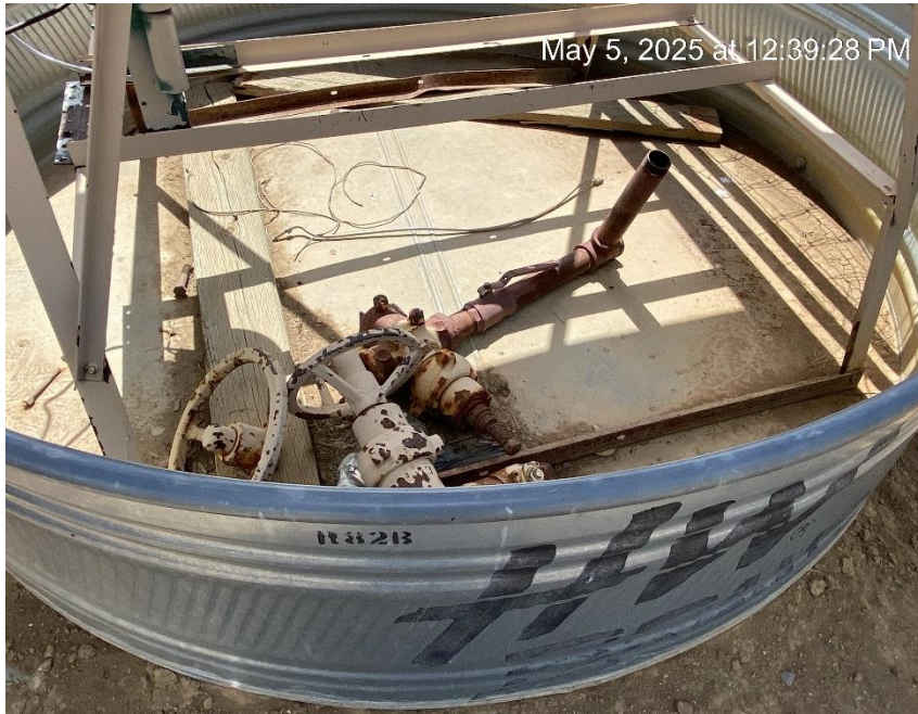
Debris. Open containment.
