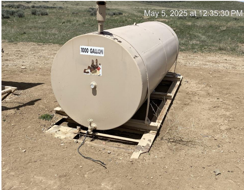
Unused equipment. Damaged label. No containment.
