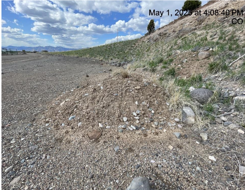
Photo # 8382 Stockpiled soils with no BMP's
