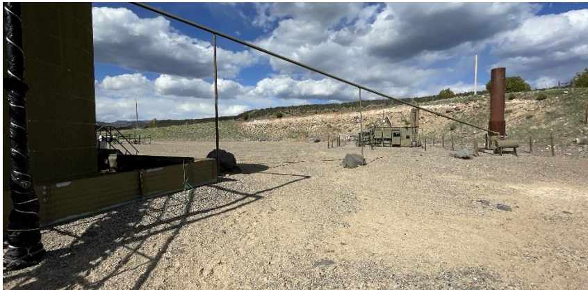
South West corner of location.
