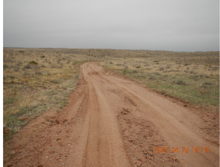
4. Repaired Access trail looking down grade from well location.
