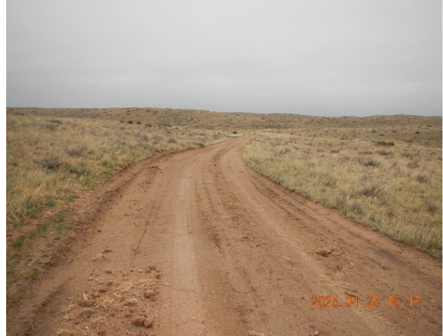
8. Repaired Access trail looking down grade from well location.
