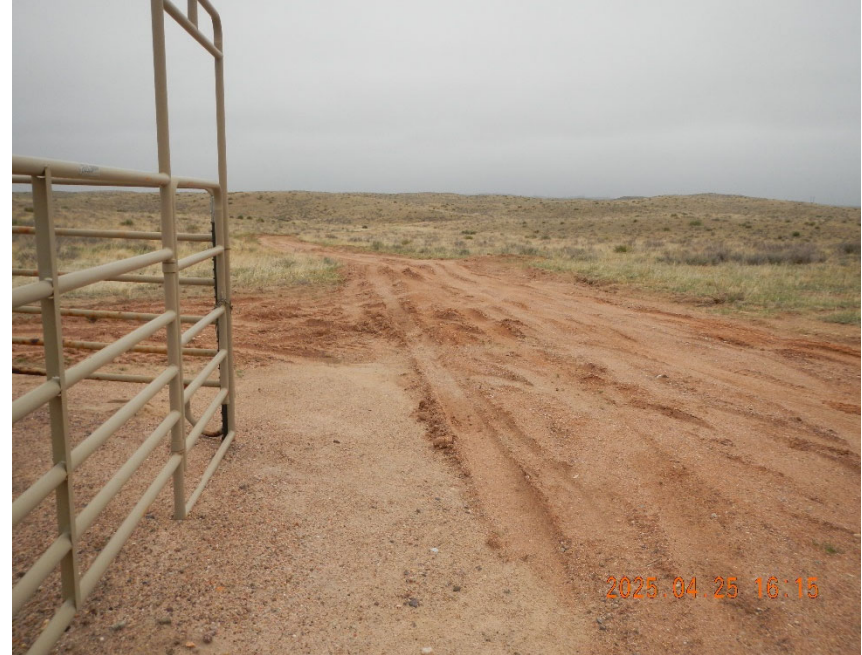
2. Photo looking down Access trail from well location.
