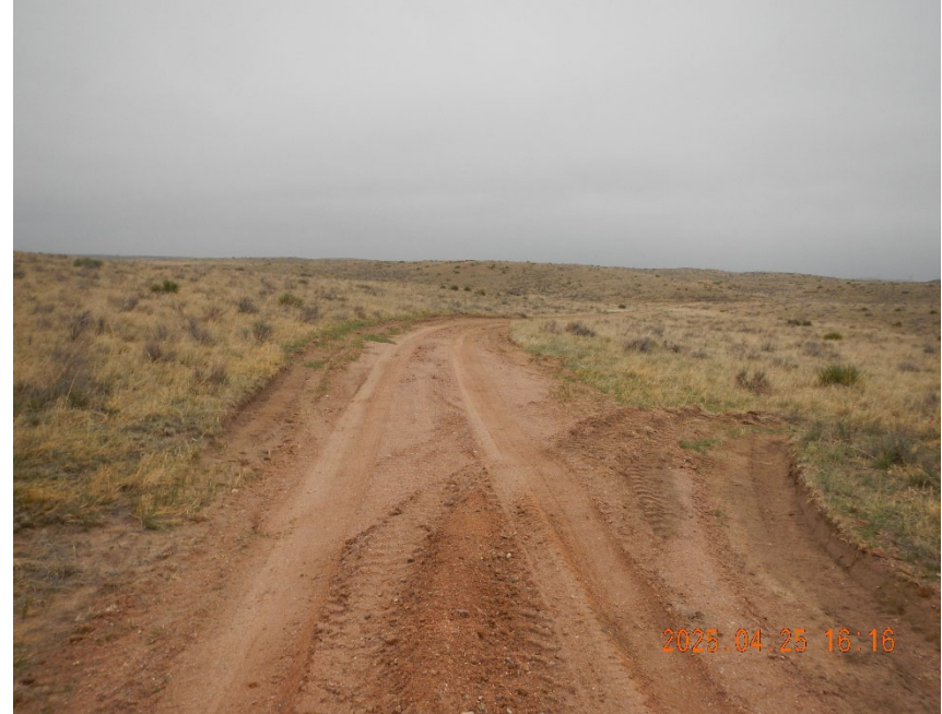
6. Repaired Access trail looking down grade from well location.
