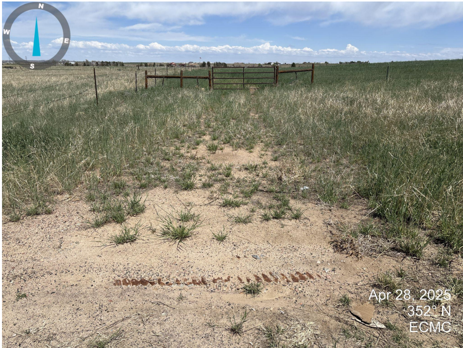
Photo 1. Looking north down access road. Culvert remains in place.
