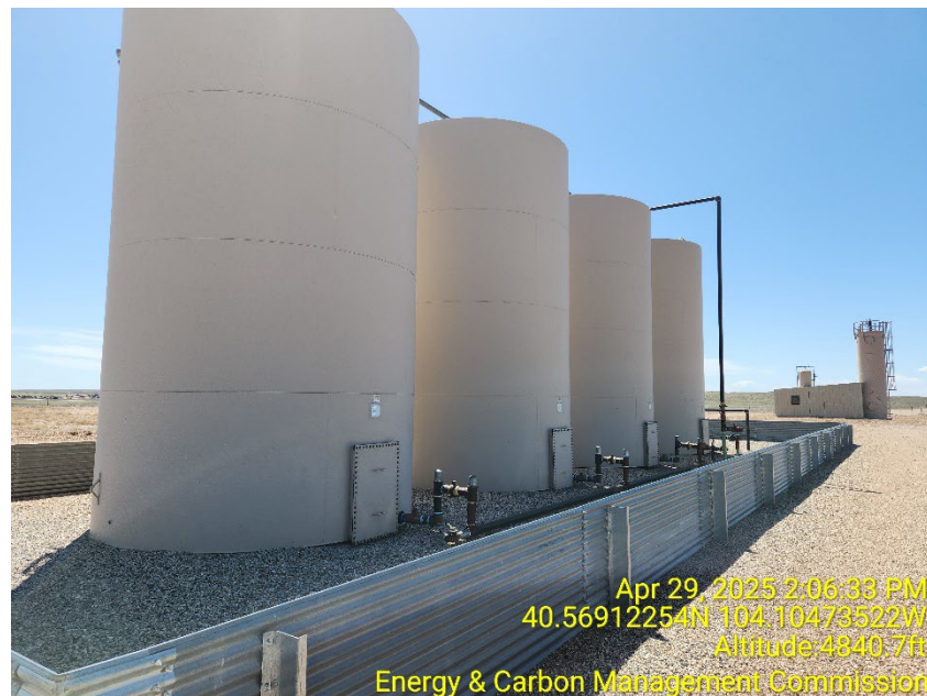
Photo 10 – Tank Battery
