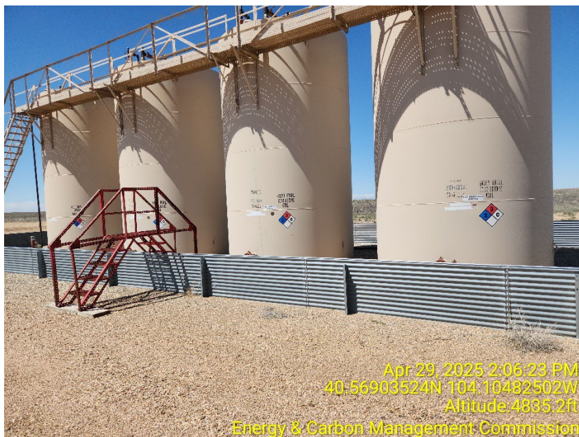
Photo 9 – Tank Battery
