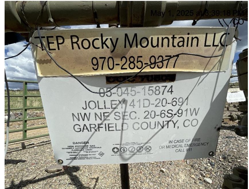
Photo # 7953 Wellhead sign lacks the public road used to access the site/not in compliance with CECMC rules
