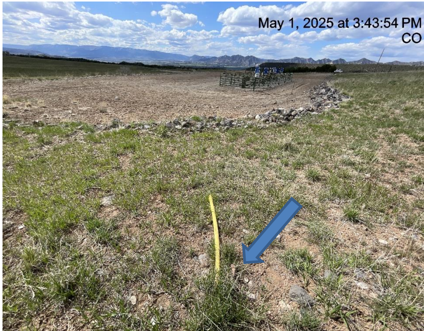
Photo # 7952 Same improperly marked deadman from a different angle
