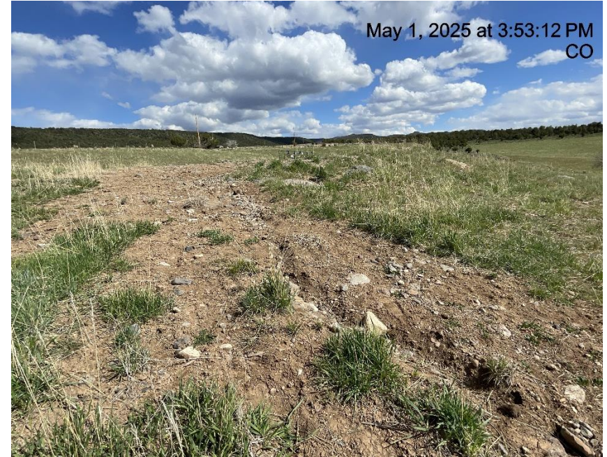
Photo # 7961 Failure to minimize erosion & the transport of sediment off location/insufficient BMP's (W/NW edge of location)
