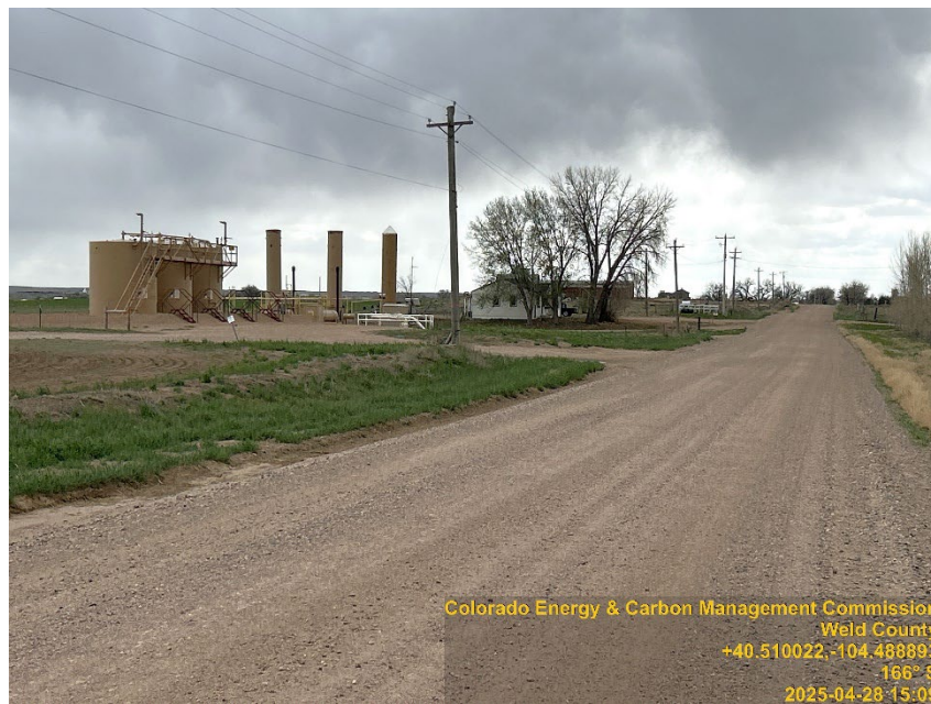
Photo #4 Foss 6-32, 6-31 Battery site Inactive | Shut-down Battery entrance
