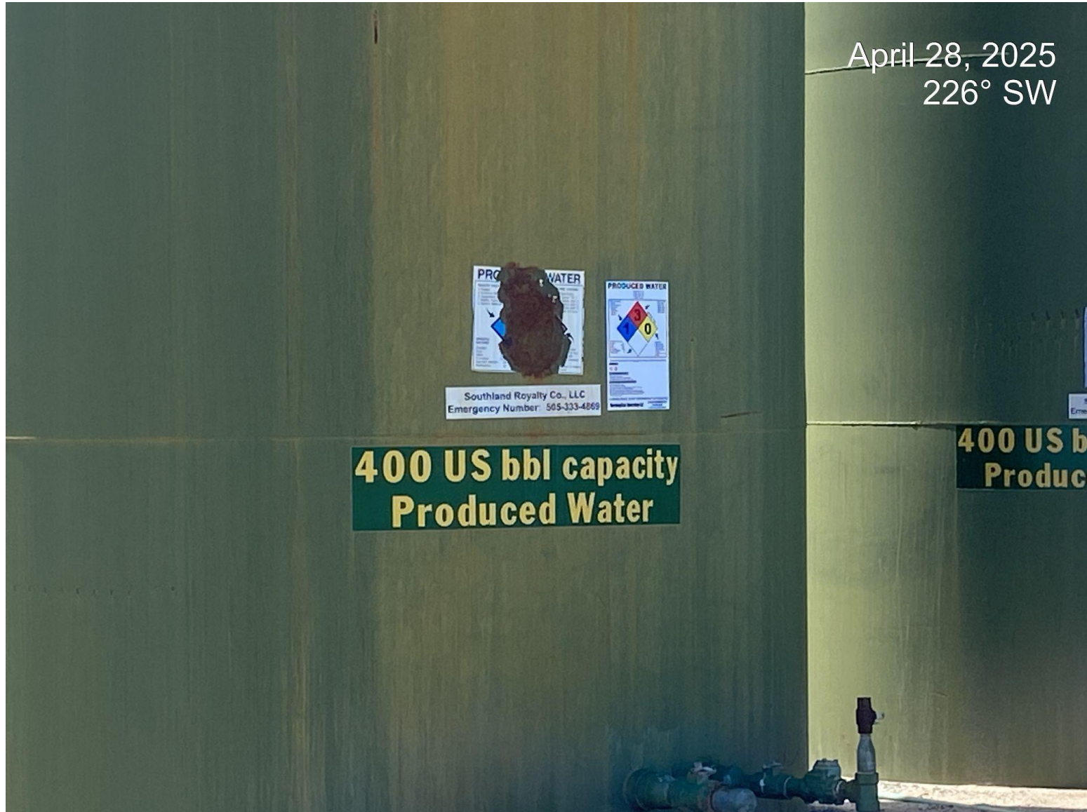
Photo 3. Produced water tank not displaying up to date operator or emergency number.
