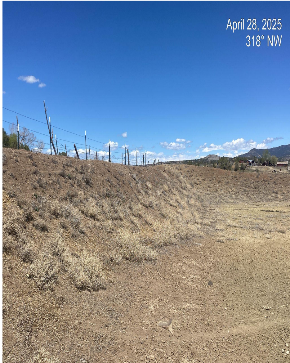
Photo 3. View of location cut slope which remains with bare soils and weedy debris.
