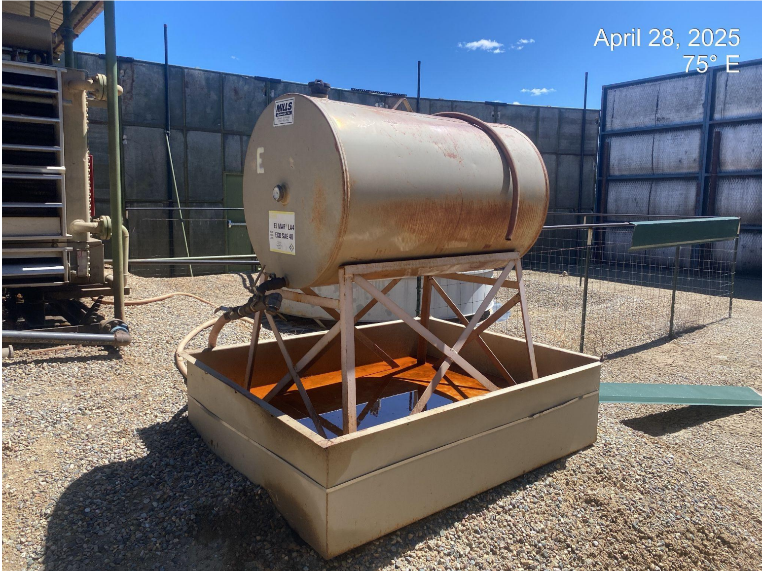
Photo 3. Chemical tank secondary containment missing wildlife BMPs/Protections.
