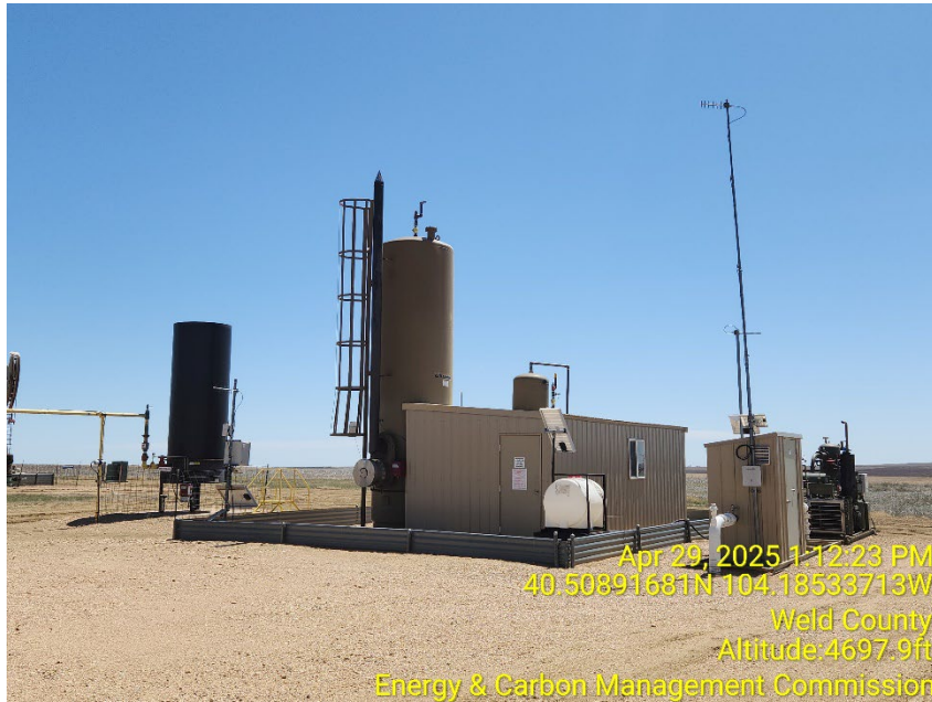
Photo 3 – Heater Treater, ECD, Gas Meter and and VRU
