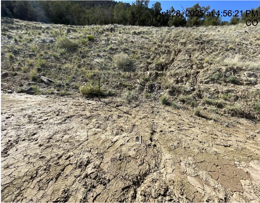
Photo # 7023 Erosion & transport of sediment on cutslope /sediment migrating onto location/insufficient BMP's
