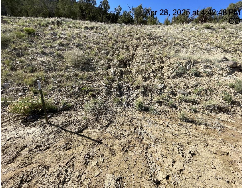
Photo # 7021 Erosion & transport of sediment on cutslope /sediment migrating onto location/insufficient BMP's
