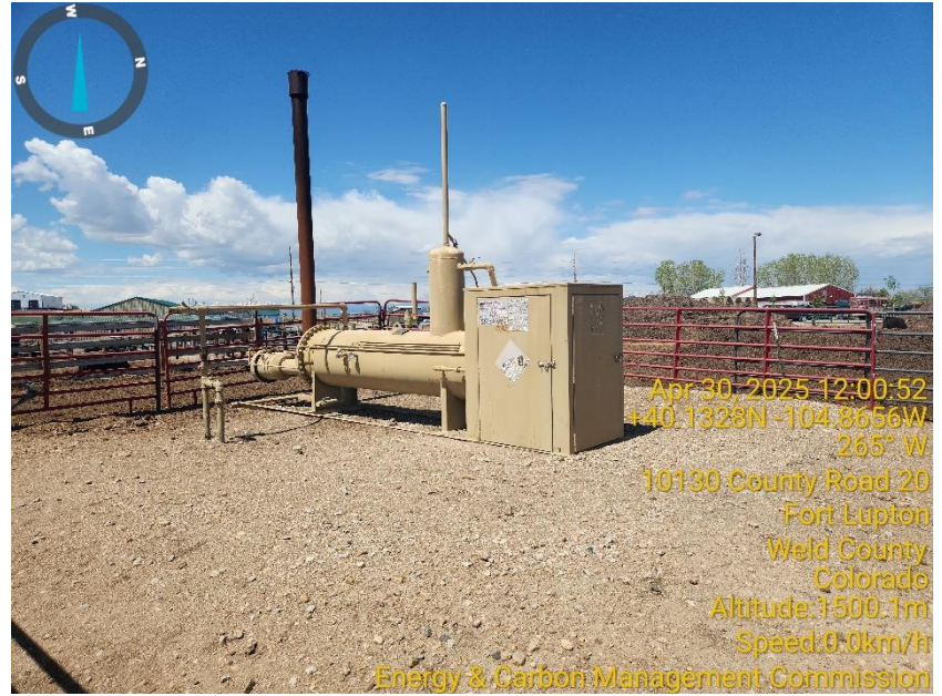
Photo 6 Horizontal heated separator.
