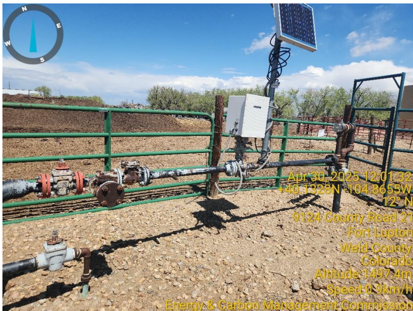
Photo 7 Gas meter run.
