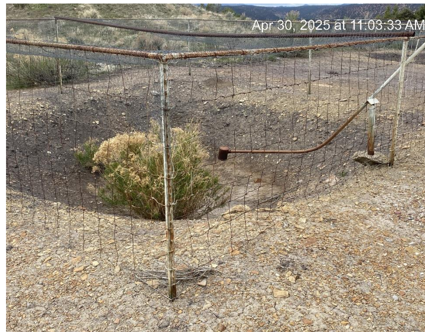
Meter run pit
