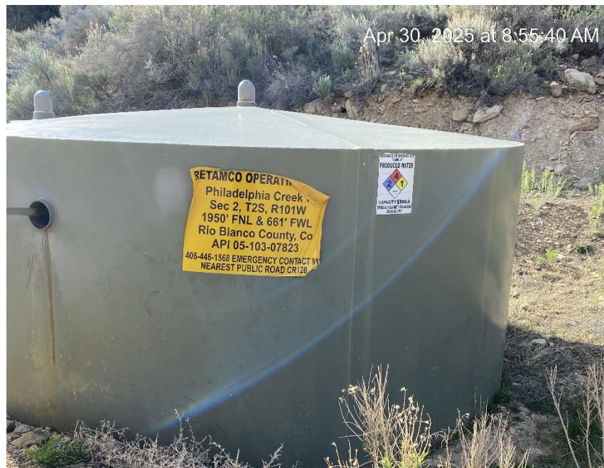
Replace damaged labels
