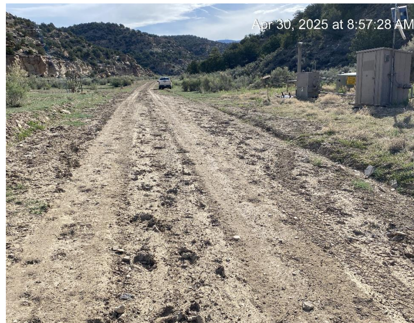
Location from Northeast entrance
