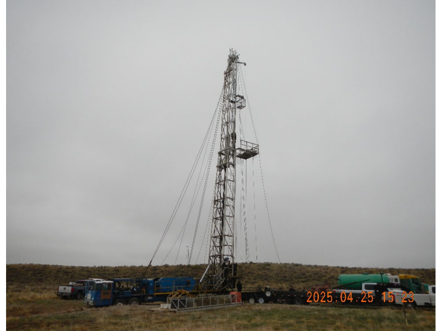
4. Well location overview with Rig over wellbore and P&A equipment on site.
