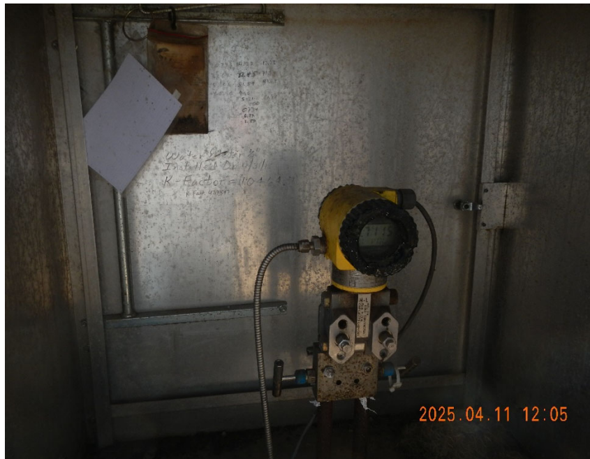
3. Gas Meter inside Flowline Meter Box.
