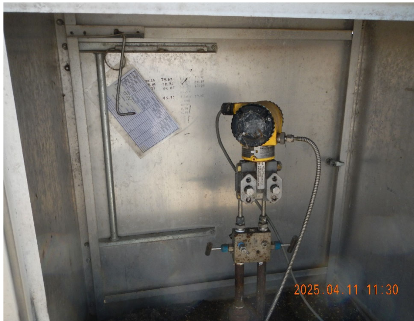
3. Gas Meter inside Flowline Meter Box.
