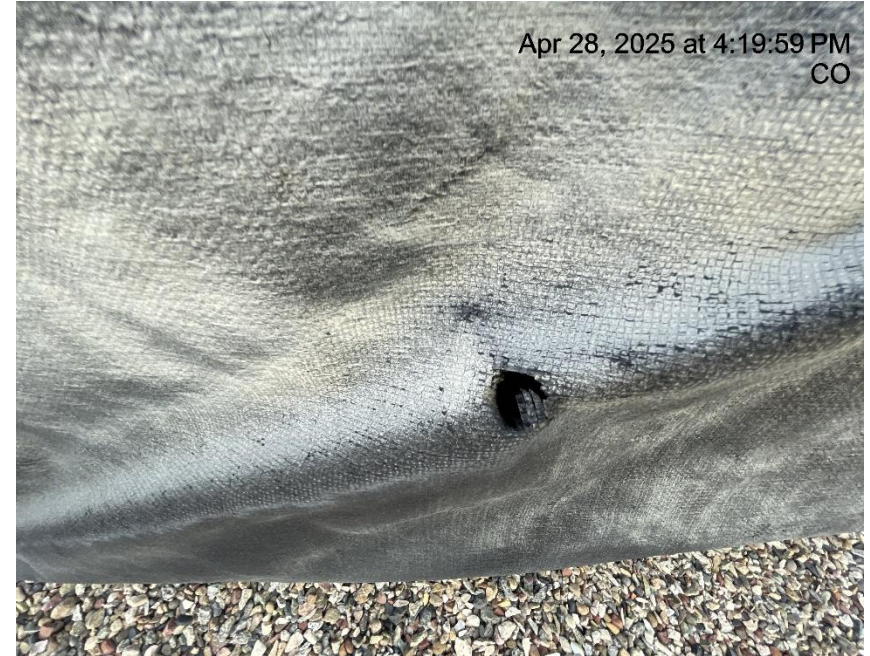
Photo # 6929 Hole in liner/liner needs maintenance
