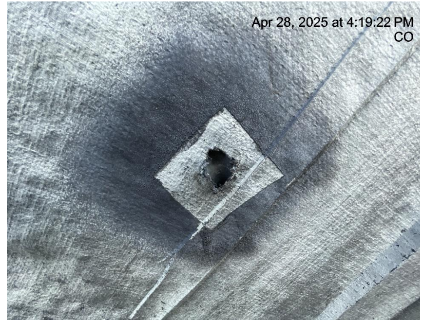
Photo # 6927 Hole in liner/liner needs maintenance
