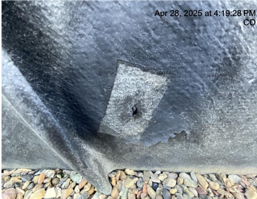
Photo # 6928 Hole in liner/liner needs maintenance
