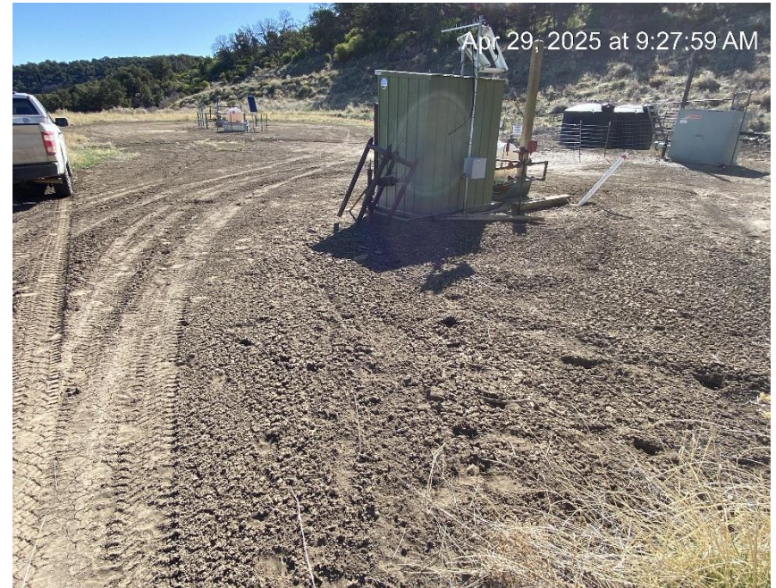
Location from Southwest entrance
