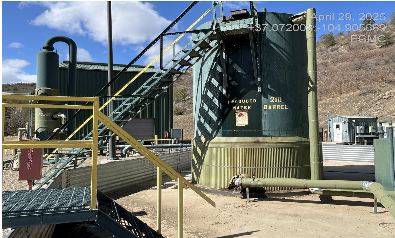
Photo 3. Facing toward the produced water tank. It appears fluids leaked out the top running down the side.
