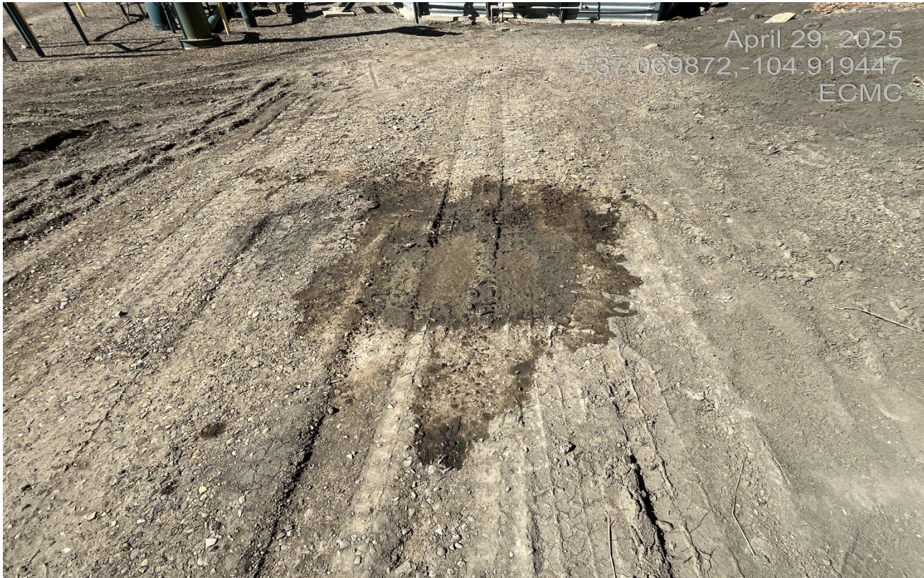
Photo 2. Oil stained soils need to be cleaned up and properly disposed..
