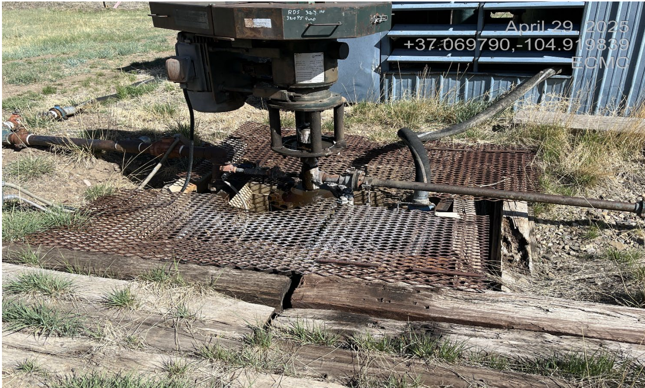
Photo 3. There is a dripping water leak at the wellhead and the grate does not fully cover the well cellar.
