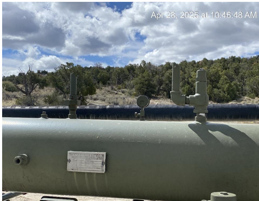
Relief vent riser caps missing
