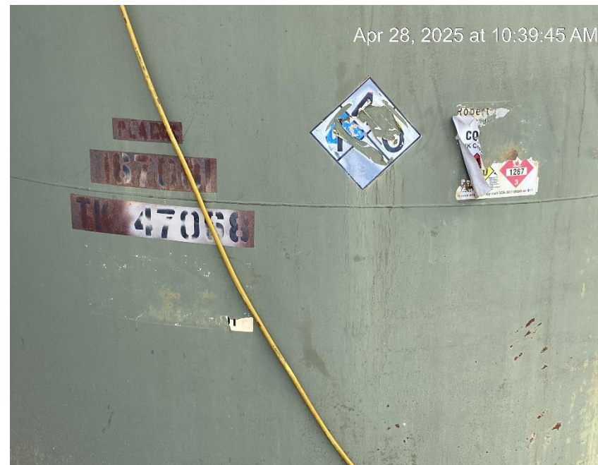
Damaged and incomplete tank label
