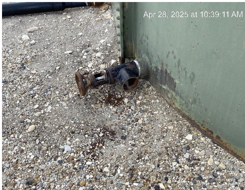
Stained soil. New soil. Open end tank valve.
