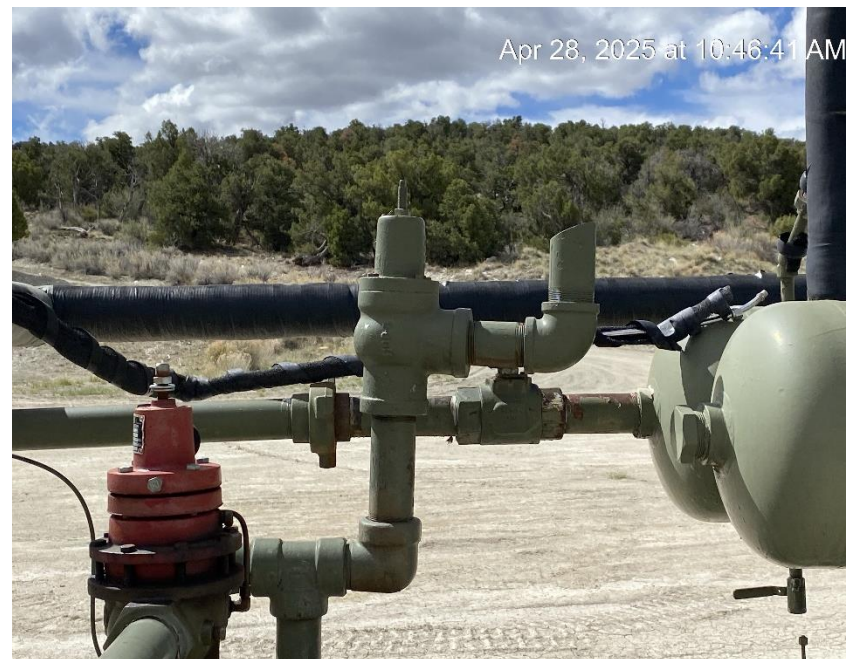
Relief vent riser cap missing
