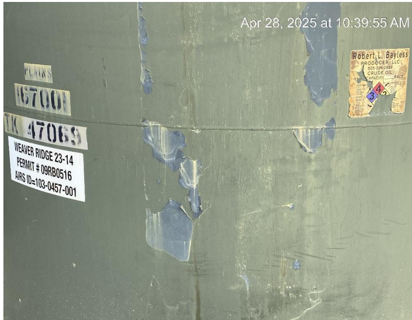
Damaged and incomplete tank label
