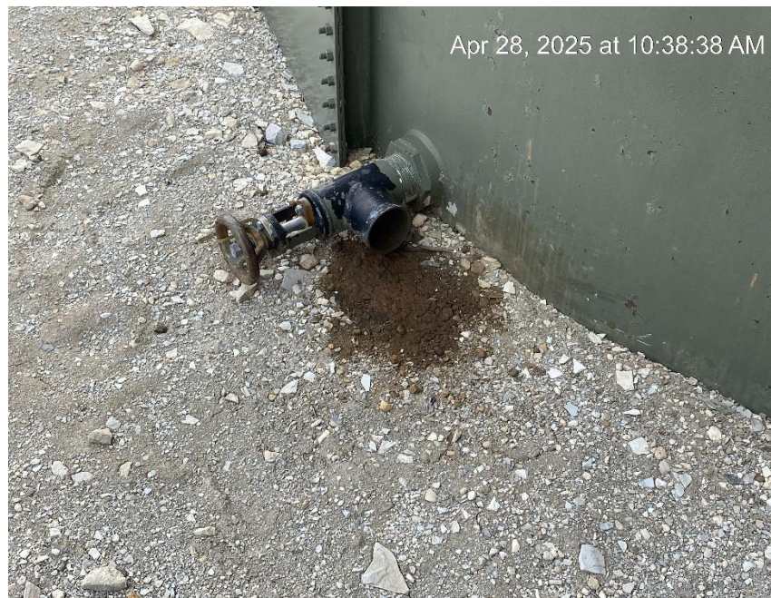
Stained soil. Open end tank valve.
