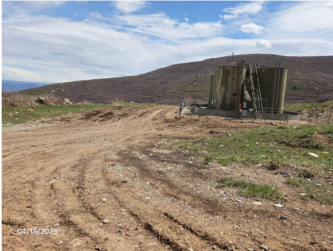
Photo 6: Photo taken from the west end of the tank battery Location, facing east. Photo shows stabilization and tracking controls show sign of disrepair; degradation/rutting observed.
