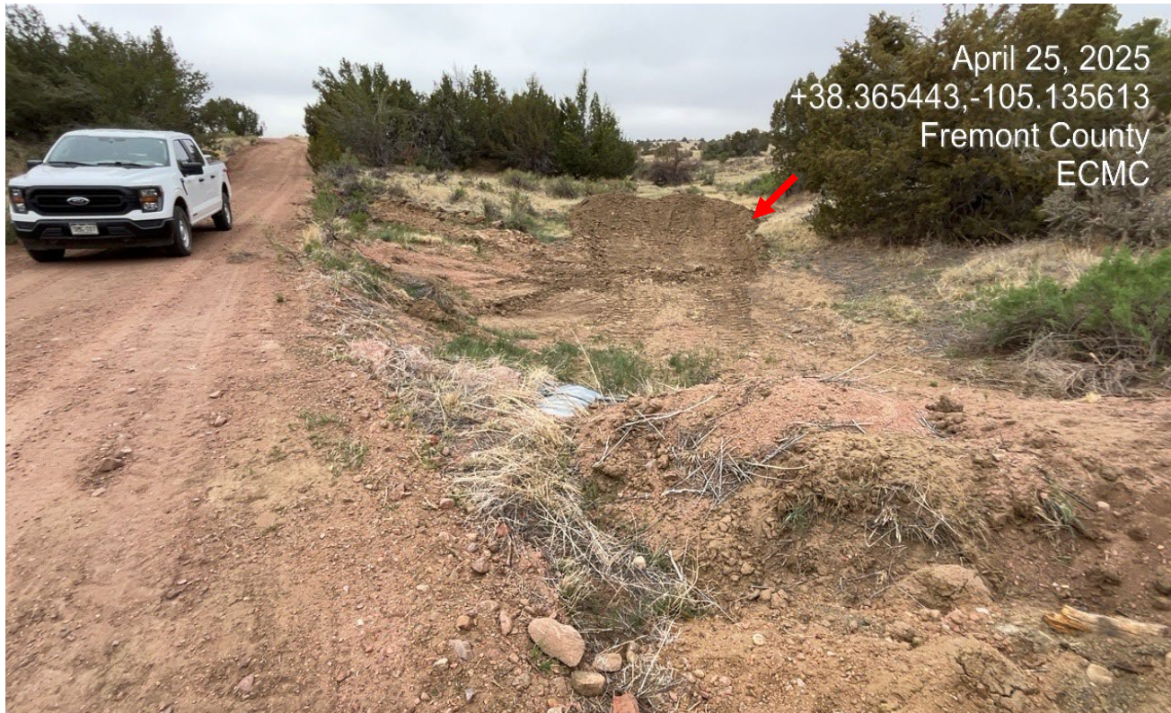
Photo 2. The sediment at the culvert outlet was pushed back in the drainage at red arrow. This material needs to be removed or slope out of the drainage so it does not wash back into the culvert.
