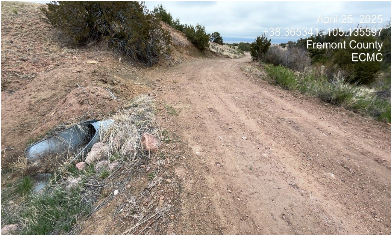
Photo 1. Facing north along the access road. There is an erosion gully along the roadside has been repaired.
