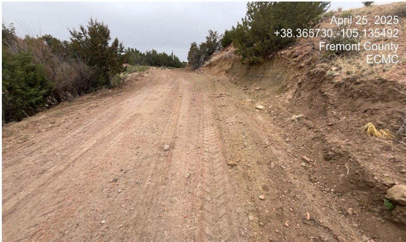
Photo 3. Facing back along the access road. The dozer cut into the embankment to fill in the erosion. The embankment cut now needs to be resloped and stabilized.
