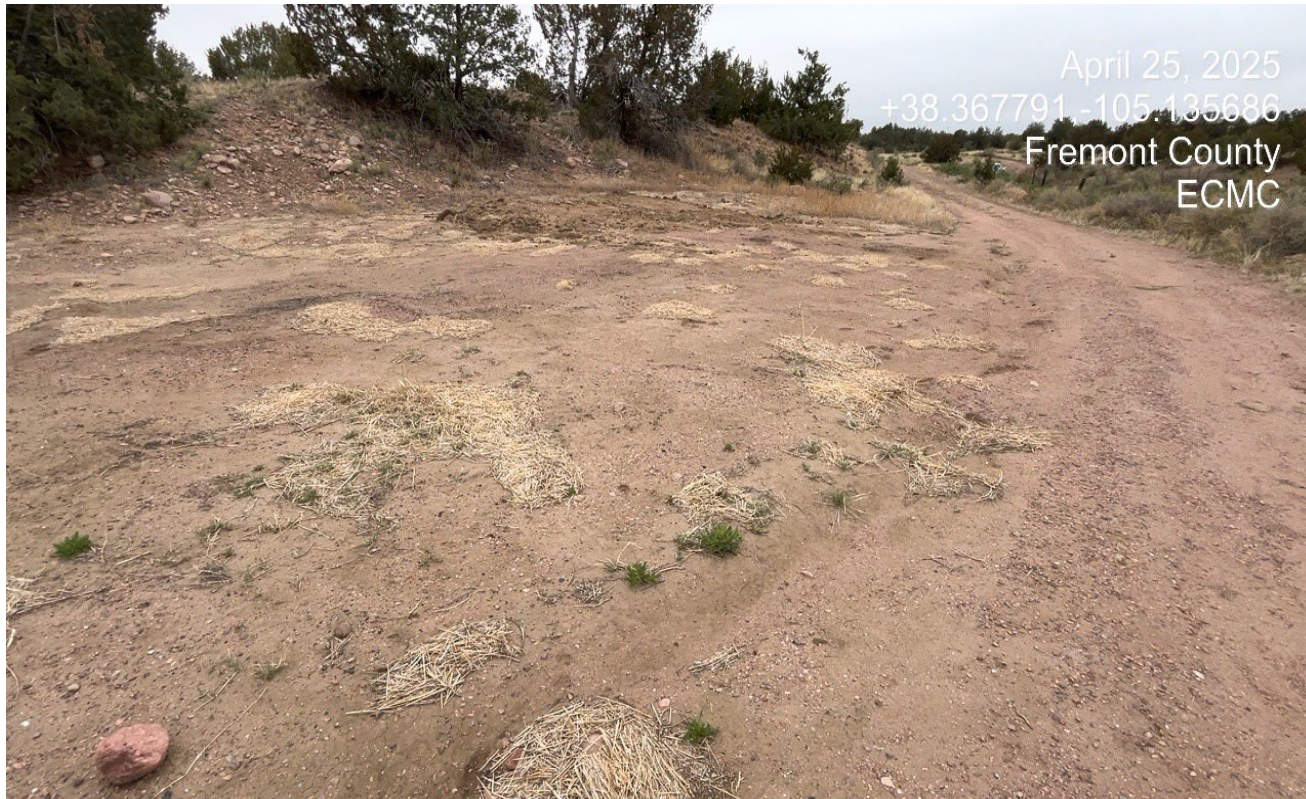
Photo 7. Facing southeast at the locations. Soils need to be cross ripped and reseeded.
