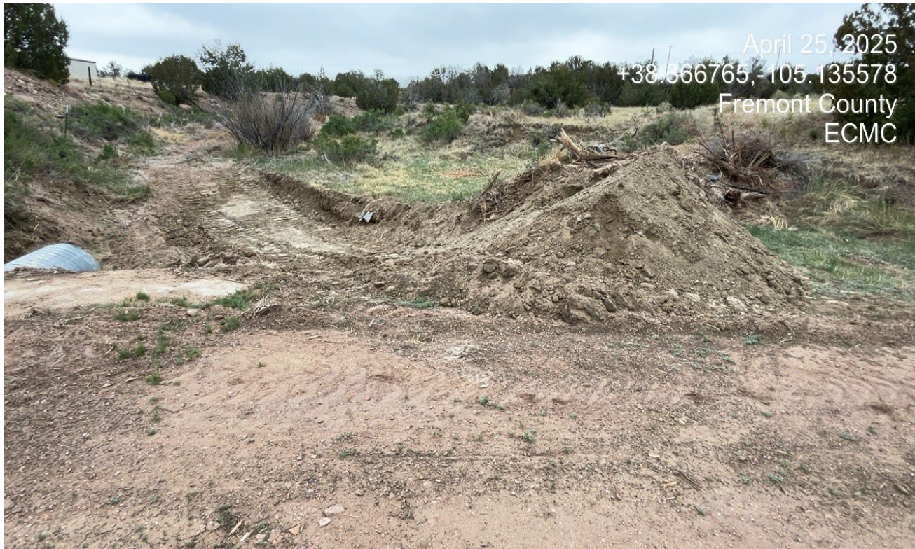
Photo 4. The culvert has been cleaned out and soil and debris is piled up along the side which needs to be removed.
