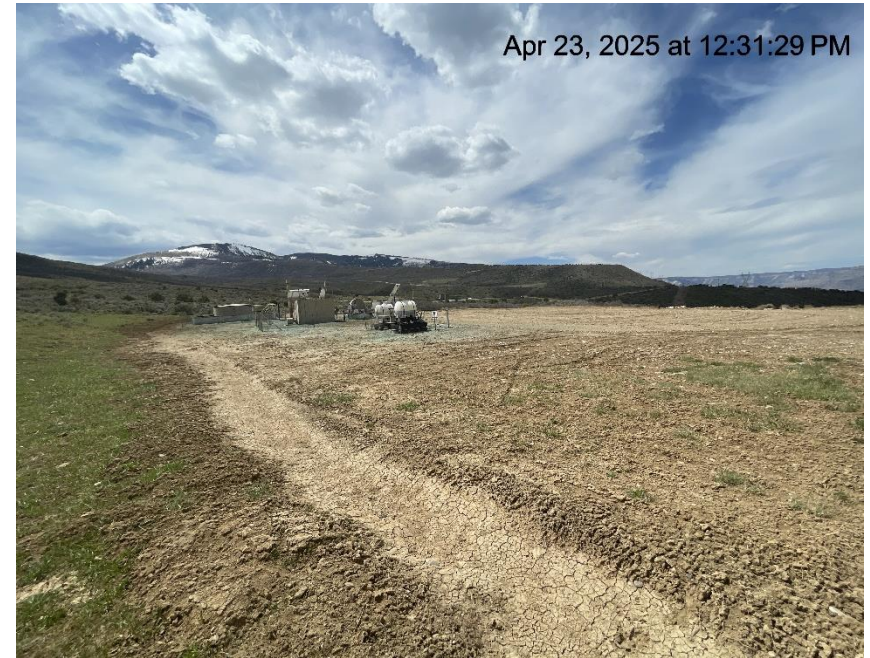
Photo # 4920 Ditch lacks any BMP's (N/NE area of location)
