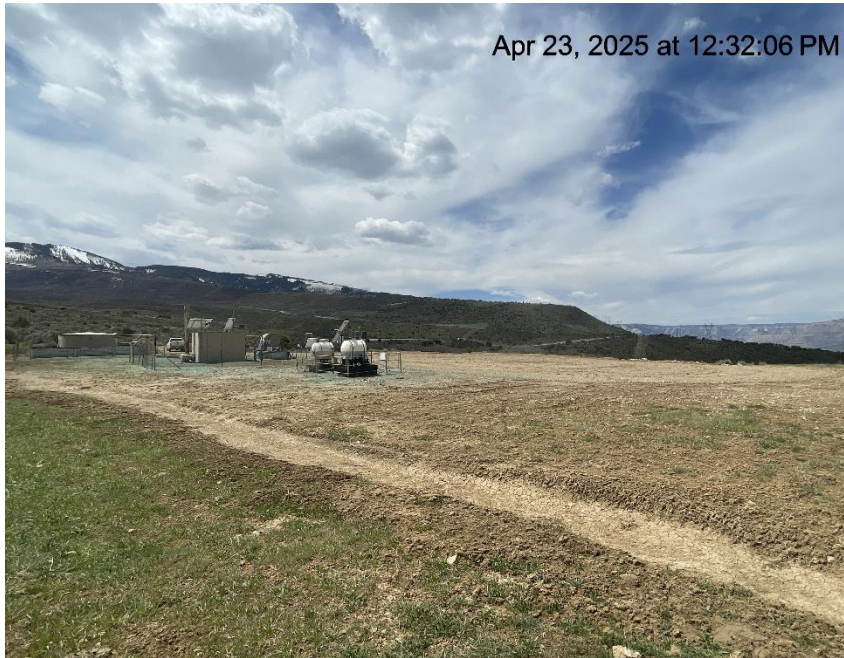
Photo # 4919 Ditch lacks any BMP's (N/NE area of location)
