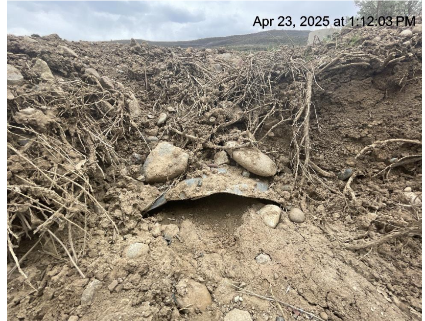
Photo # 5057 Culvert on lease road near entrance to location needs maintenance
