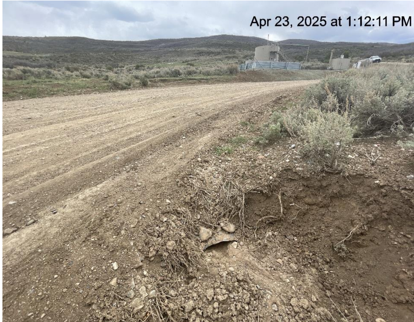
Photo # 5056 Culvert on lease road near entrance to location needs maintenance
