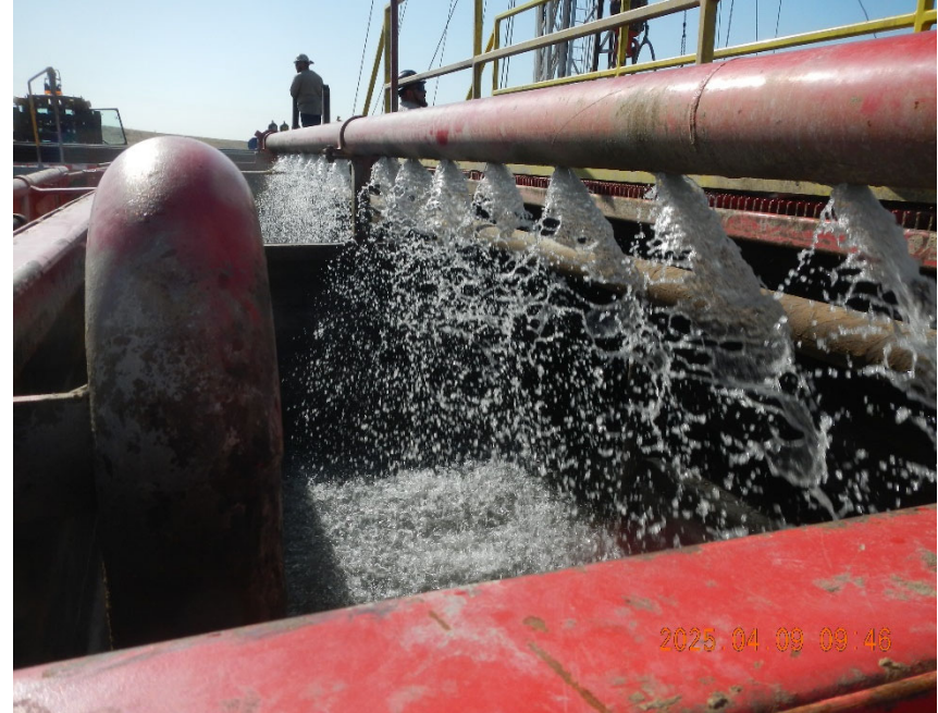
4. Water returns to surface establishing circulation to surface in preparation to place cement into wellbore.
