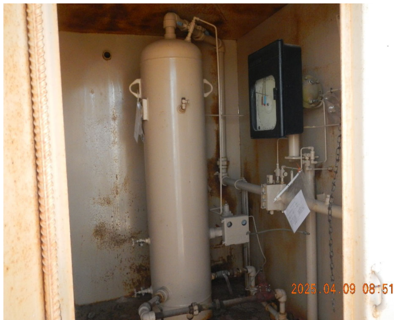
5. View of vertical separator inside steel shed.
