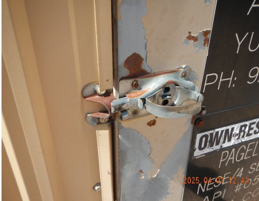
5. Broken meter shed door handle. Door is jammed shut.
