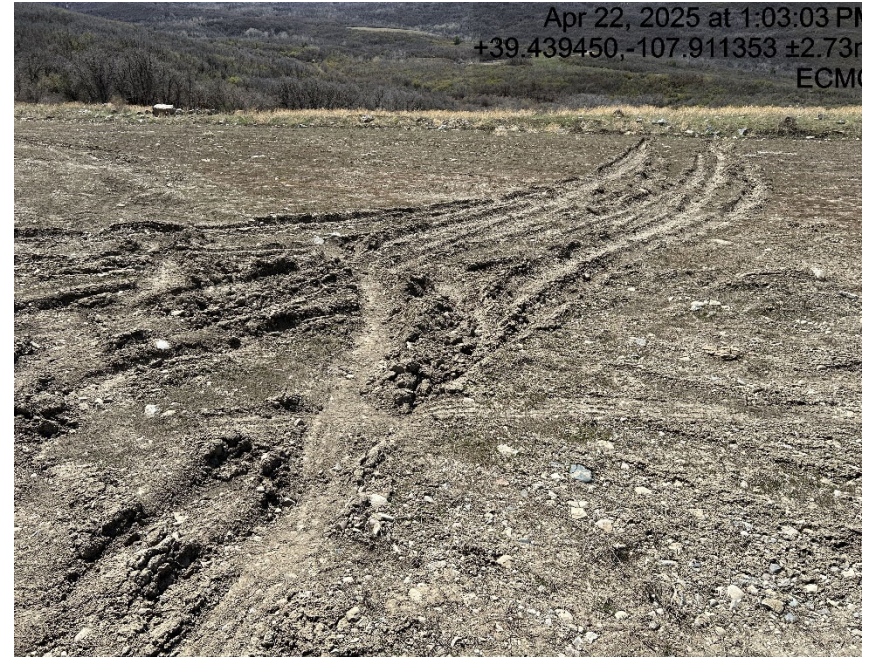
Lack of stabilization/compaction
