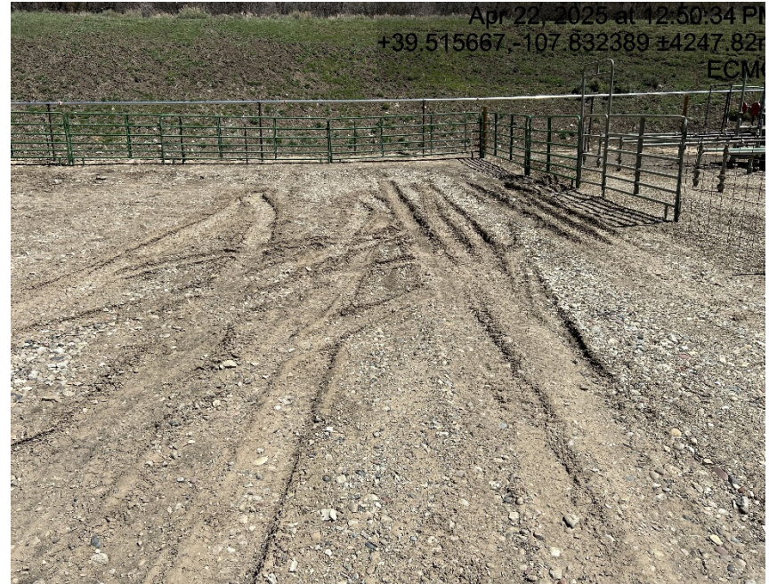
Lack of stabilization/compaction
