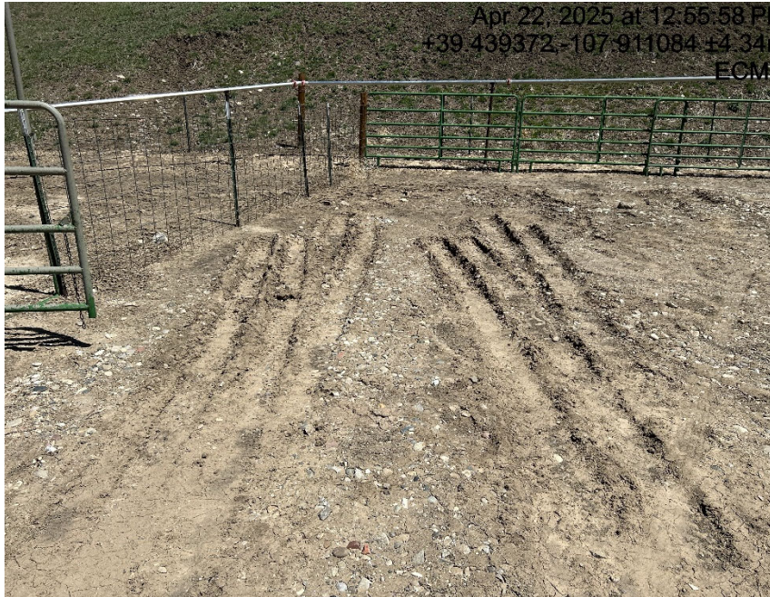
Lack of stabilization/compaction
