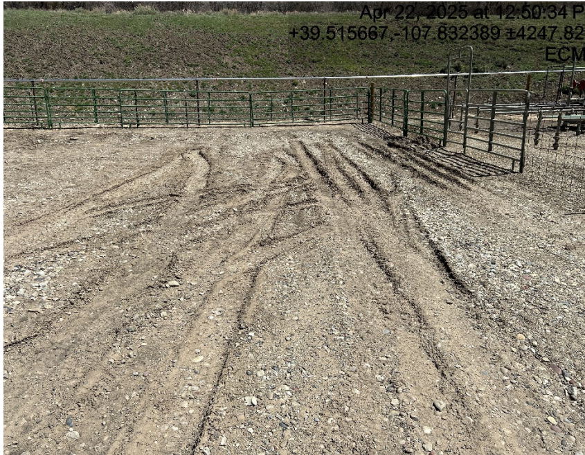
Lack of stabilization/compaction
