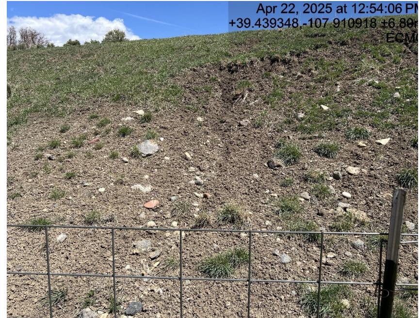
Erosion on cut slope by tank battery
