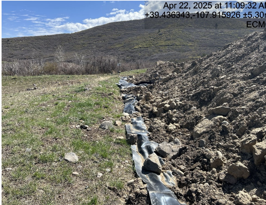
BMP's failing
