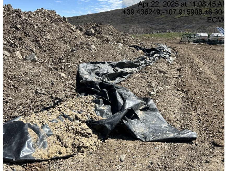
BMP's failing
