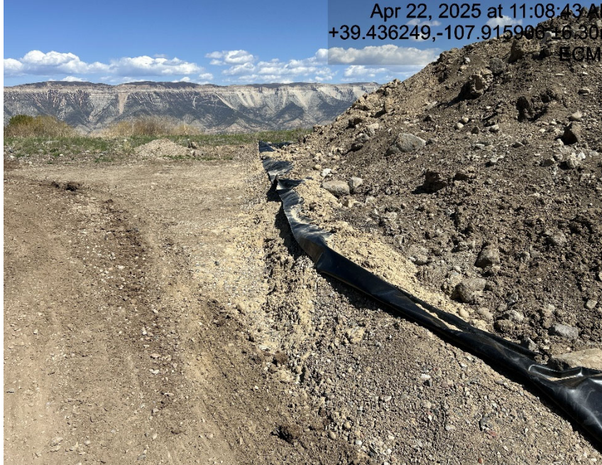
BMP's failing
