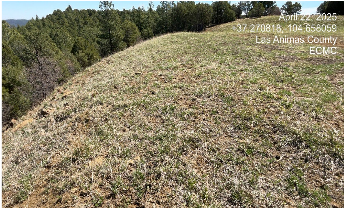
Photo 4. Facing toward the fill slope which is stabilized with perennial vegetation.
