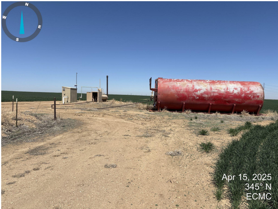
Photo 3. Looking north down the east side of the location. Bucket of oil has been removed. Produced water tank without secondary containment remains on location.
