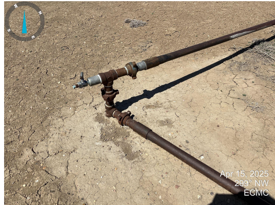
Photo 4. Looking at the joint between produced water tank and separator. Does not appear to be leaking. Some soil may have been removed around the joint.
