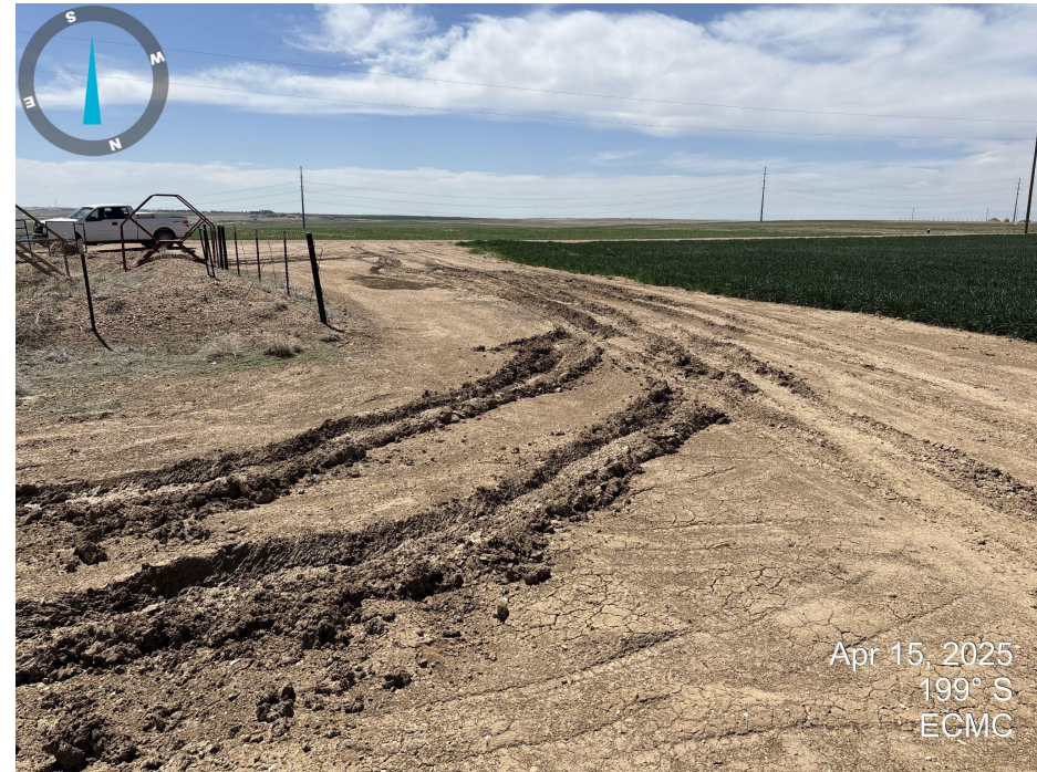
Photo 6. Deep ruts in the access road to the west of the tank battery.
