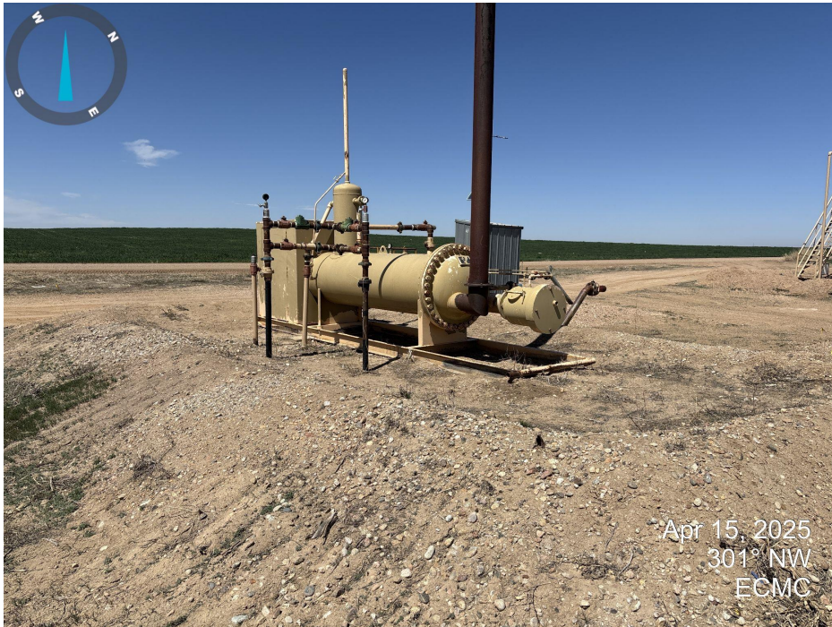
Photo 9. South side of separator at the sank battery. Tank battery location has been mowed. Weeds have been removed from secondary containment. Trash has been removed from around separator.
