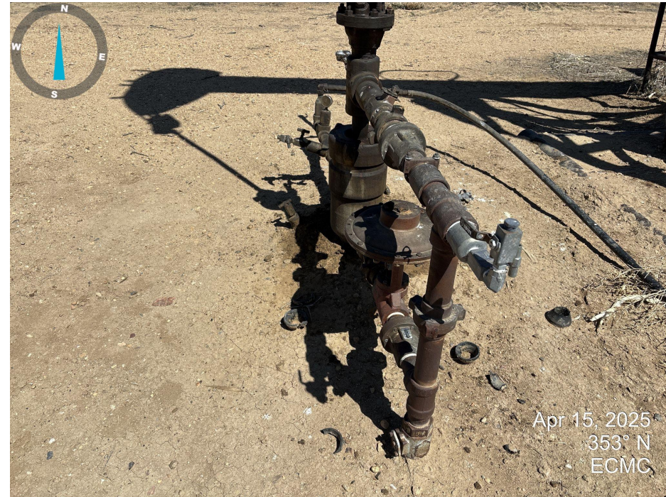
Photo 8. West side of wellhead. See photo 7 comments.
