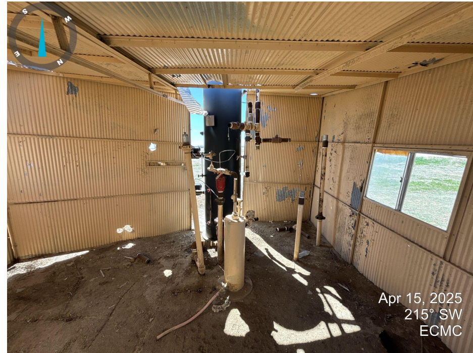
Photo 8. Inside of southern separator shed. Stained soil remains around separator.
