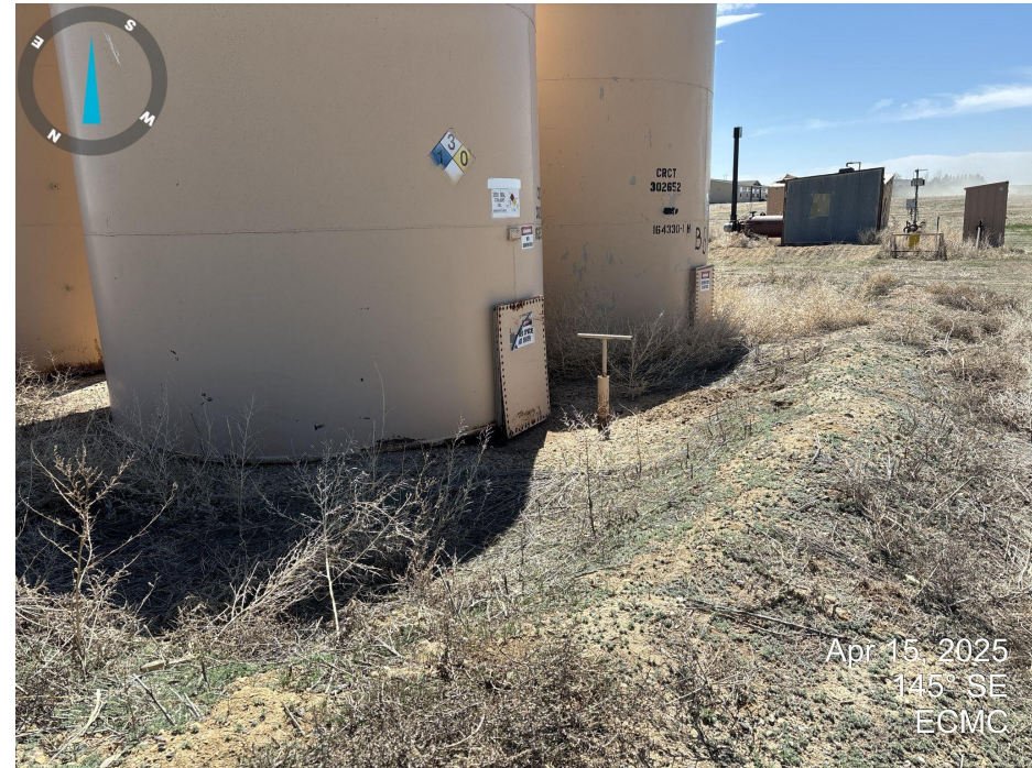
Photo 2. Looking south across the west side of the tank battery. Undesirable weeds such as Kochia and Russian Thistle are present inside of secondary containment.
