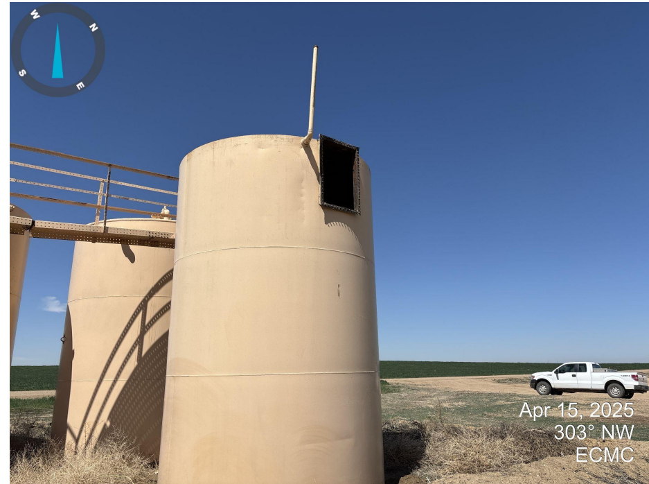
Photo 4. The eastern tank has an open inspection hatch. Birds were observed entering the hatch at the time of inspection.
