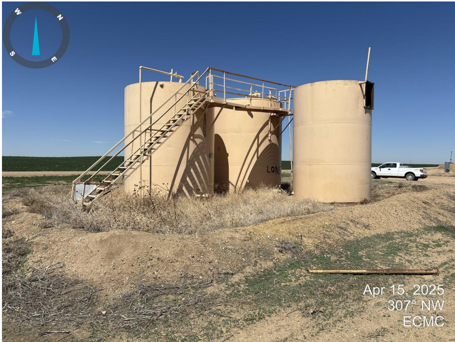
Photo 3. Looking northwest at the east side of the tank battery. Undesirable weeds inside of secondary containment. Unused equipment remains on site.
