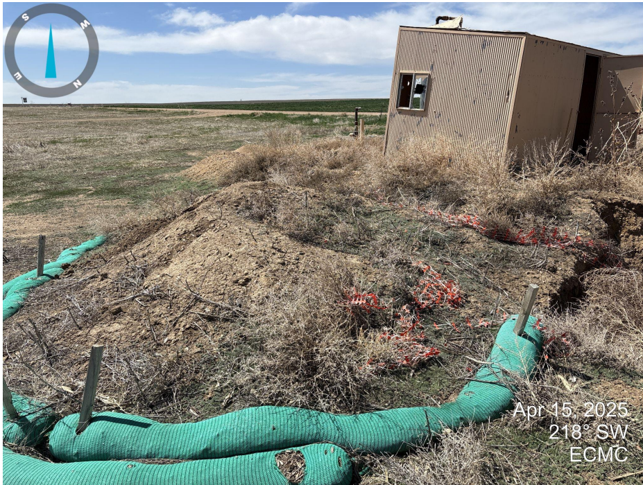
Photo 7. Soil pile and stormwater BMPs remain on location.
