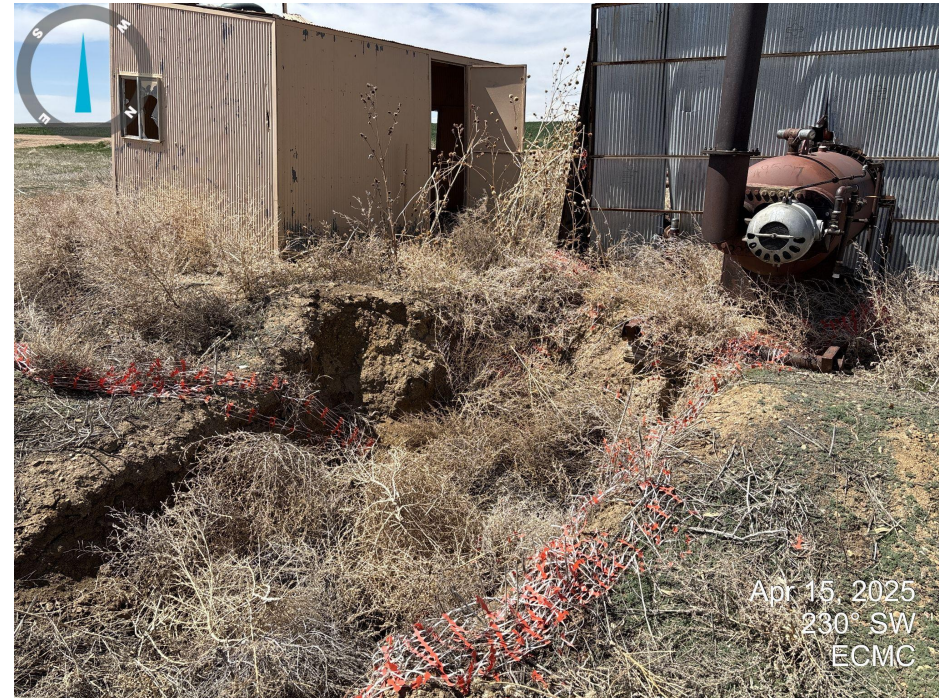
Photo 6. Open excavation remains. Fence is improperly installed. Undesirable weedy vegetation such as Kochia and Russian Thistle is present around the sheds.
