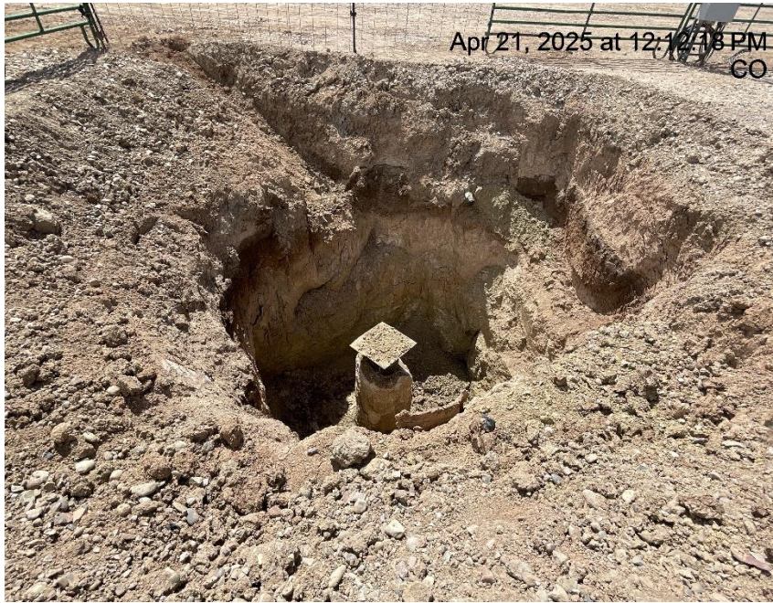
Photo # 3566 Excavated area around wellhead lacks wildlife egress/wildlife hazard
