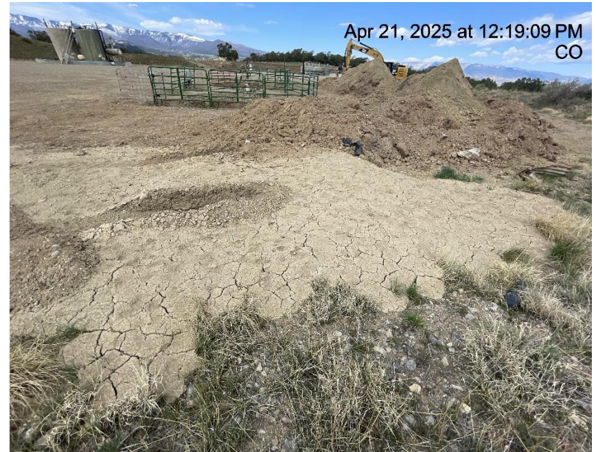
Photo # 3595 Stockpiled soils with no BMP's/not in compliance with CECMC Stormwater rules
