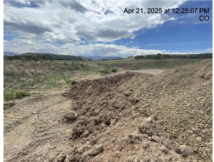
Photo # 3589 Insufficient BMP's around stockpiled soils/BMP not constructed in accordance with good engineering practices/not in compliance with CECMC Stormwater rules
