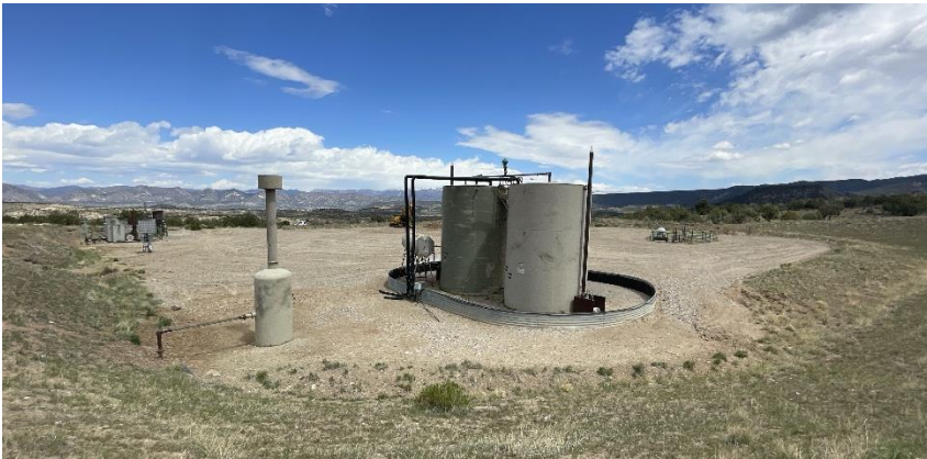
South West corner of location.
