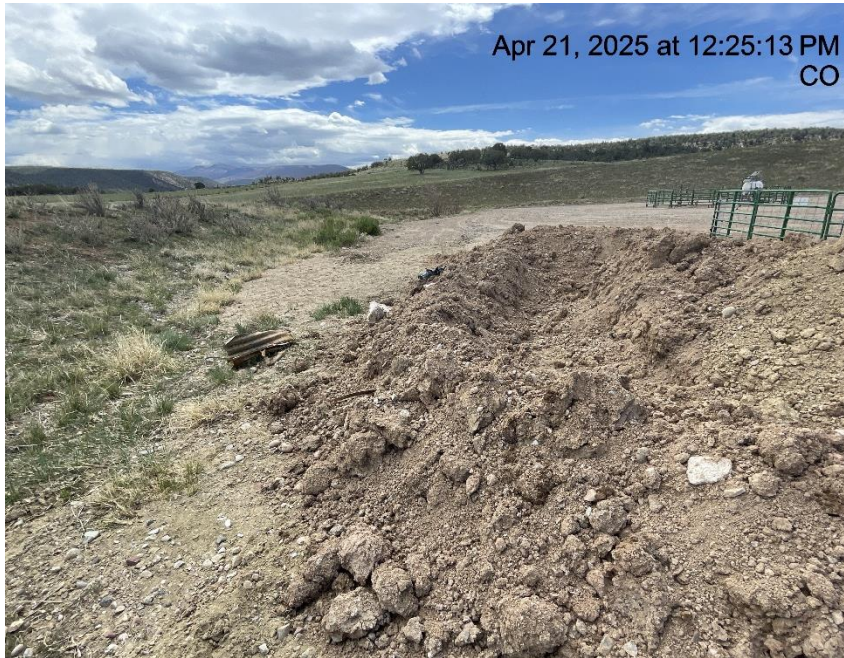
Photo # 3590 Insufficient BMP's around stockpiled soils/BMP not constructed in accordance with good engineering practices/not in compliance with CECMC Stormwater rules
