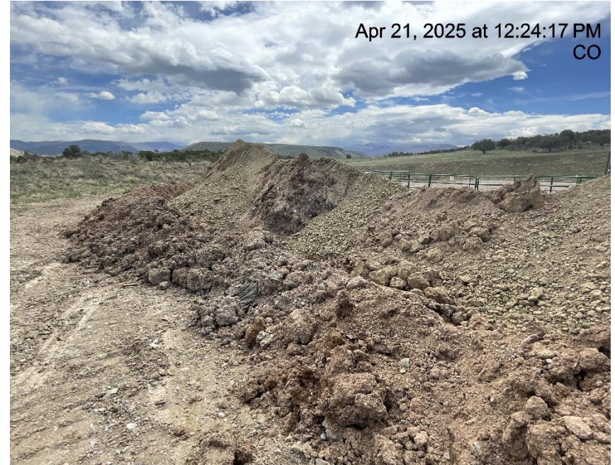
Photo # 3587 Insufficient BMP's around stockpiled soils/BMP not constructed in accordance with good engineering practices/not in compliance with CECMC Stormwater rules
