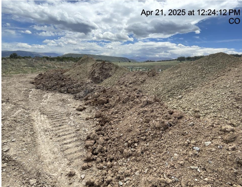
Photo # 3586 Insufficient BMP's around stockpiled soils/BMP not constructed in accordance with good engineering practices/not in compliance with CECMC Stormwater rules
