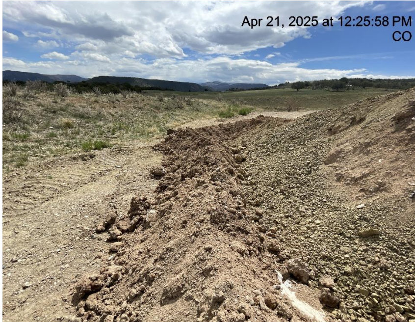
Photo # 3588 Insufficient BMP's around stockpiled soils/BMP not constructed in accordance with good engineering practices/not in compliance with CECMC Stormwater rules
