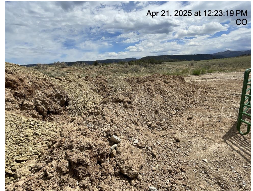
Photo # 3591 Insufficient BMP's around stockpiled soils/BMP not constructed in accordance with good engineering practices/not in compliance with CECMC Stormwater rules
