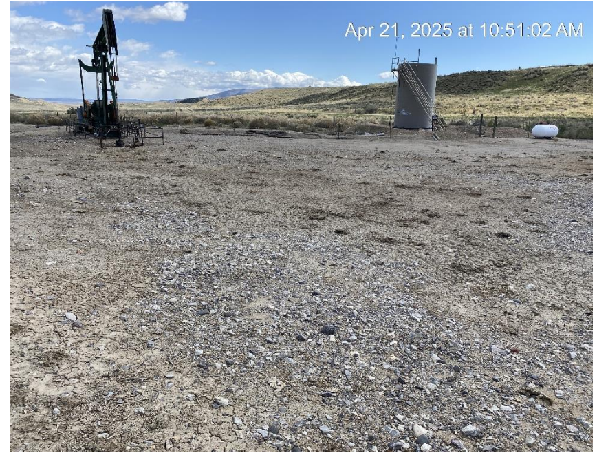
Location from South corner
