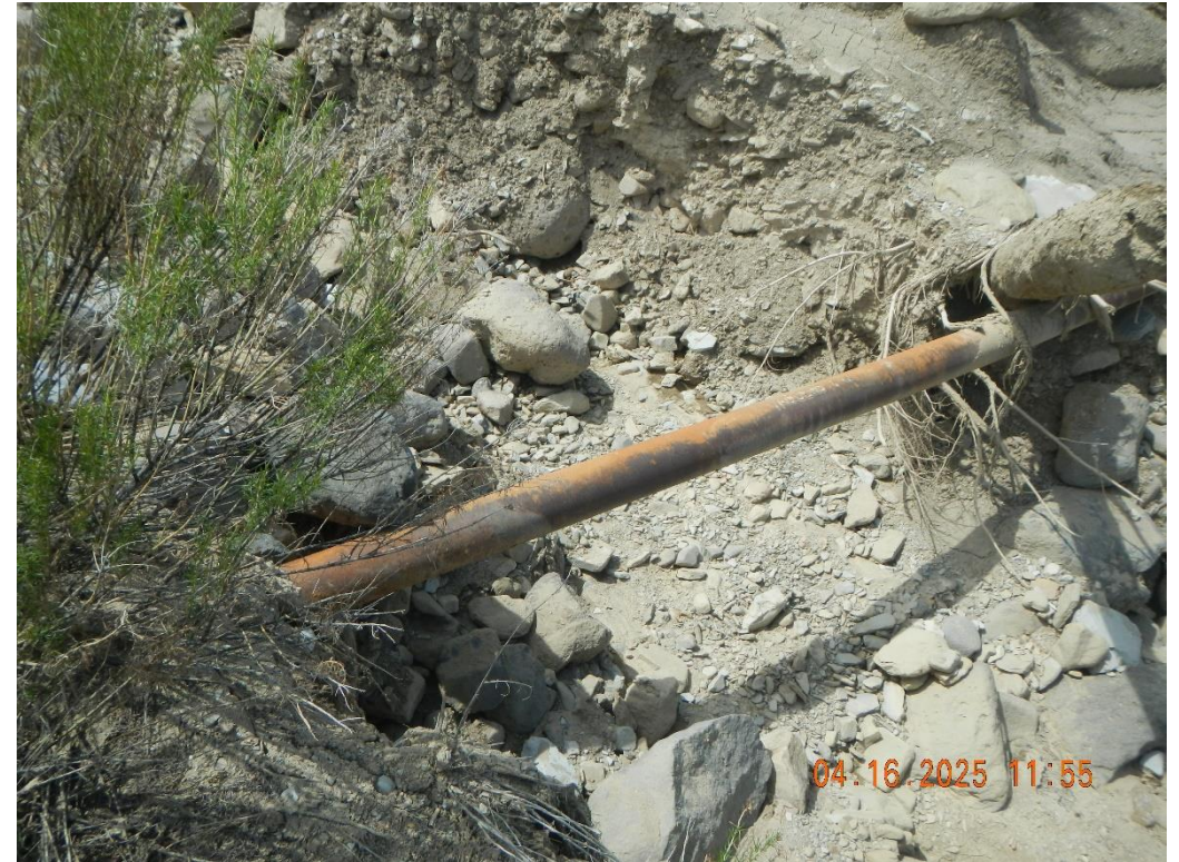
Photos from 4/16/2025 Vaquero welded on pipe
