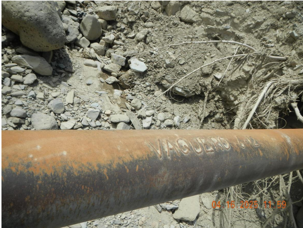
Photos from 4/16/2025 Vaquero welded on pipe
