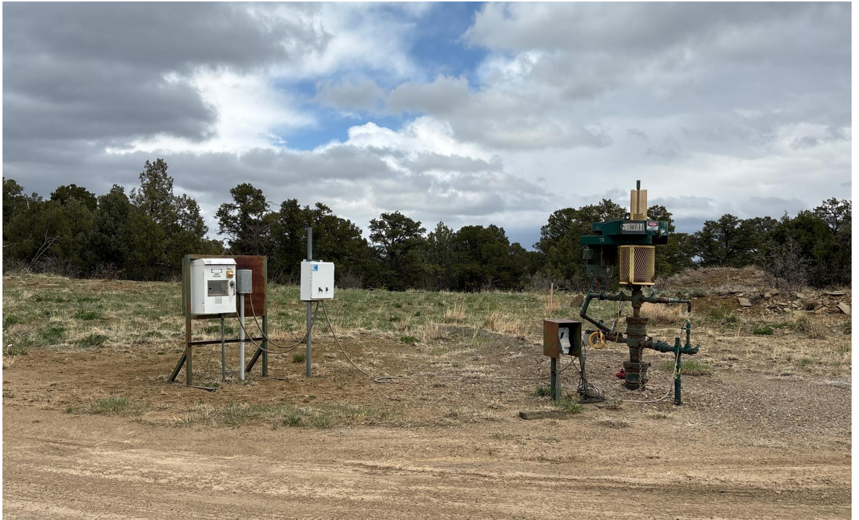
PHOTO 4: TR WELLHEAD AND EQUIPMENT.
