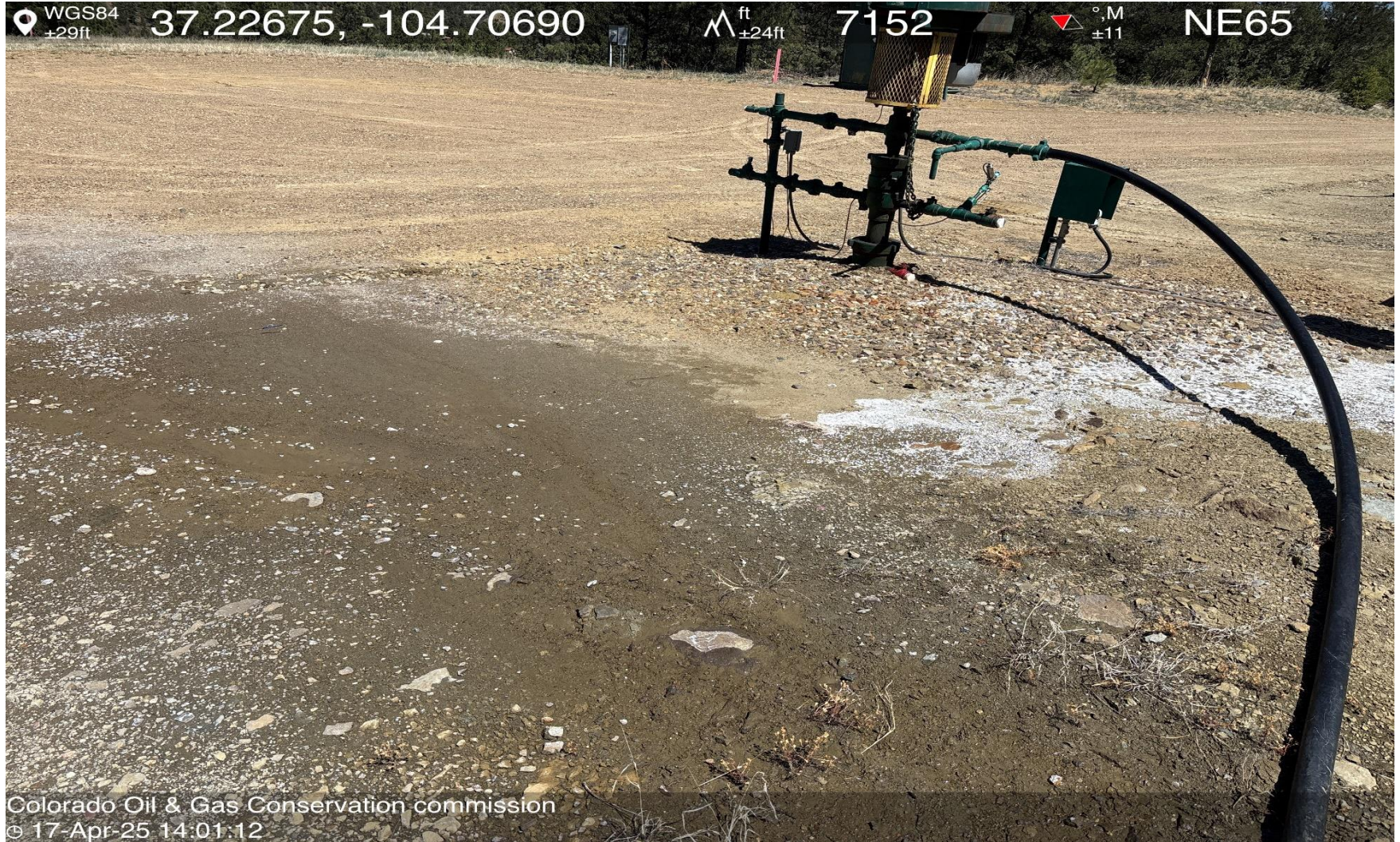
PHOTO 6: WHITE CHALKY MINERAL BUILDUP ON GROWNED AROUND WELLHEAD AND SPILL INDICATES THAT THESE CONDITION HAS BEEN PRESENT FOR AN EXTENDED TIME. Conduct maintenance on equipment, cleanup stained material and review self inspection processes. COMPLY WITH RULE 1002,(2).D CA DATE 4/28/2025.
