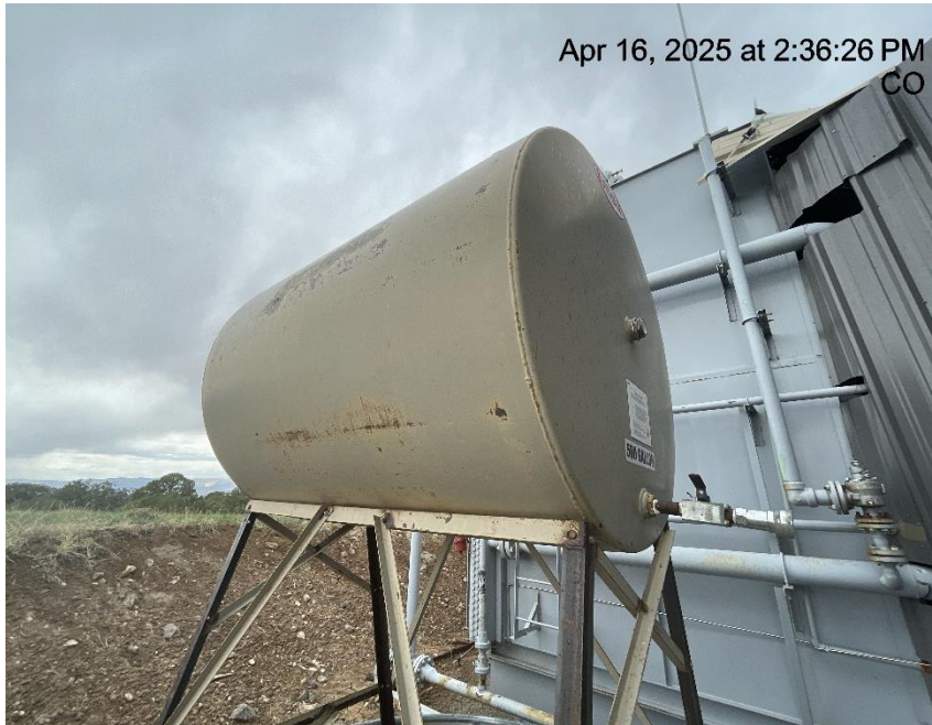
Photo # 2205 Glycol tank label lacks required information /not in compliance with CECMC rules
