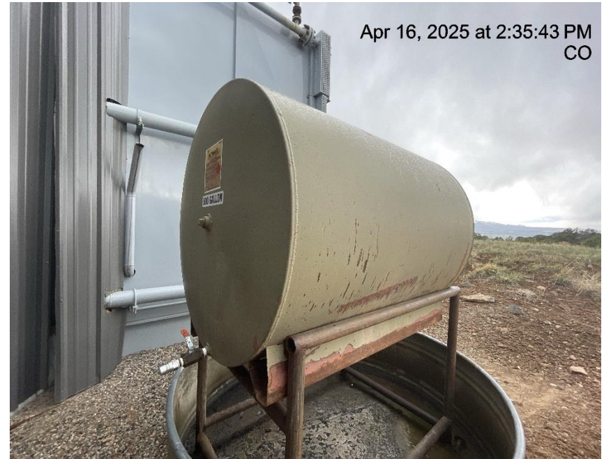
Photo # 2202 Methanol tank label lacks required information/not in compliance with CECMC rules
