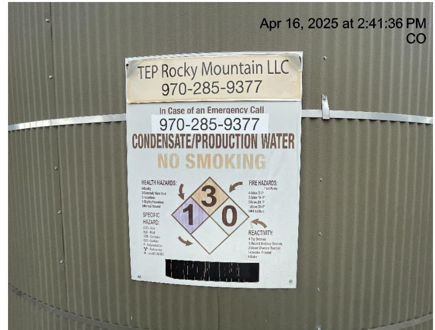
Photo # 2212 Tank label weathered & damaged/some required information is illegible/not in compliance with CECMC rules
