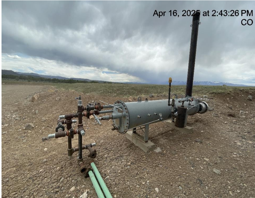
Photo # 2213 Unused equipment (additionally there's open ended piping on the unused equipment which constitutes a wildlife hazard)
