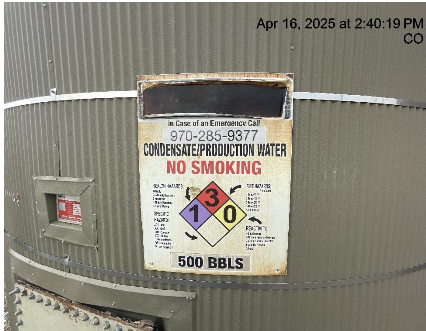
Photo # 2211 Tank label weathered & damaged/some required information is illegible/not in compliance with CECMC rules
