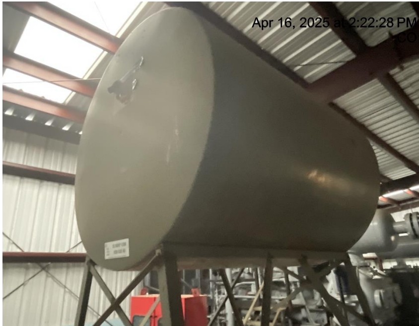
Photo # 2209 Compressor oil tank label lacks required information/not in compliance with CECMC rules
