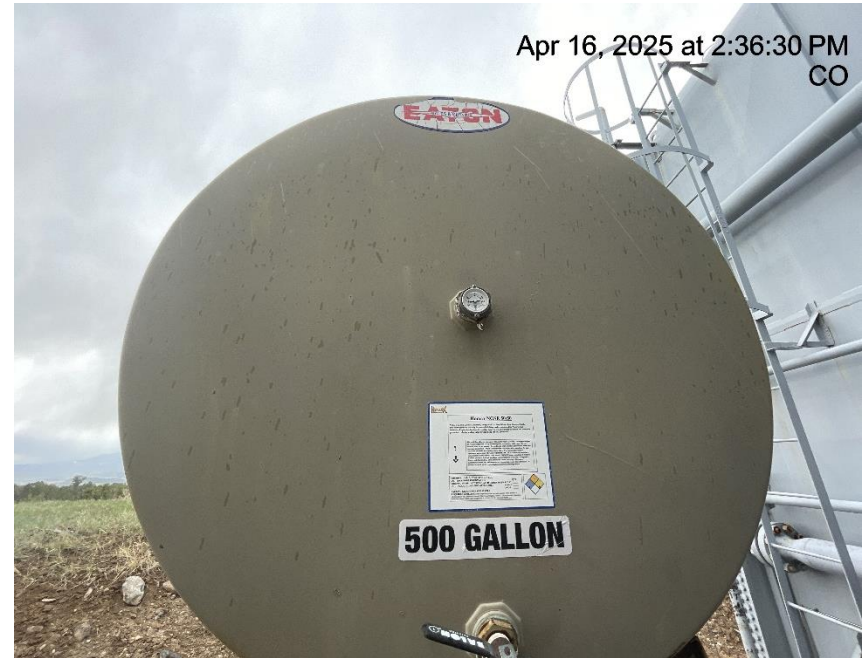
Photo # 2204 Glycol tank label lacks required information/not in compliance with CECMC rules
