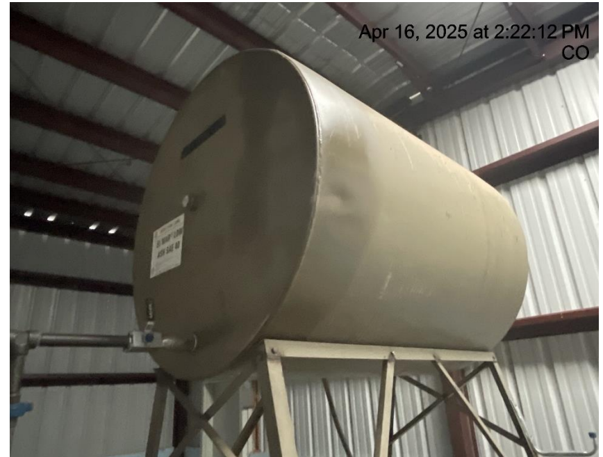
Photo # 2208 Compressor oil tank label lacks required information/not in compliance with CECMC rules
