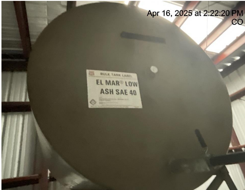
Photo # 2207 Compressor oil tank label lacks required information/not in compliance with CECMC rules
