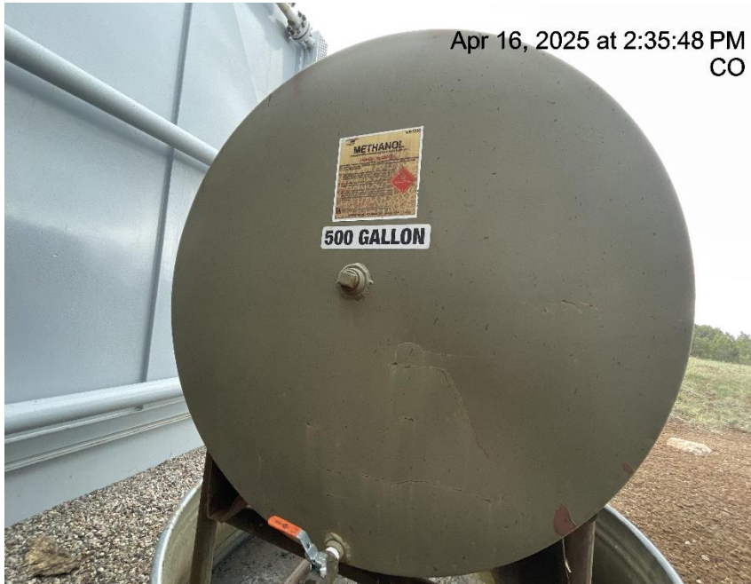
Photo # 2201 Methanol tank label lacks required information/not in compliance with CECMC rules
