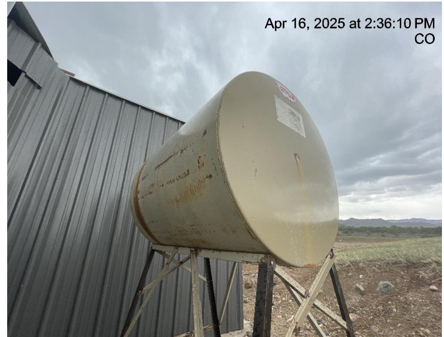
Photo # 2206 Glycol tank label lacks required information /not in compliance with CECMC rules
