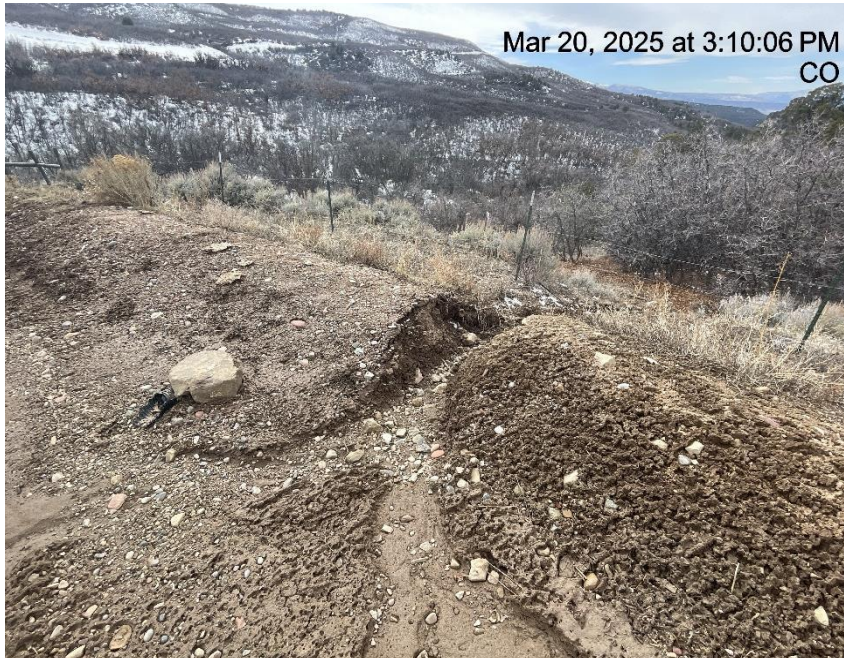
Photo # 6259 From inspection 708906071 conducted on 03/20/2025 Erosion & transport of sediment off location /berm needs maintenance
