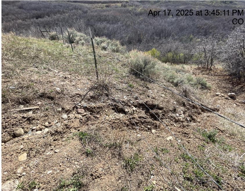
Photo # 2897 Erosion & transport of sediment off location /berm needs maintenance
