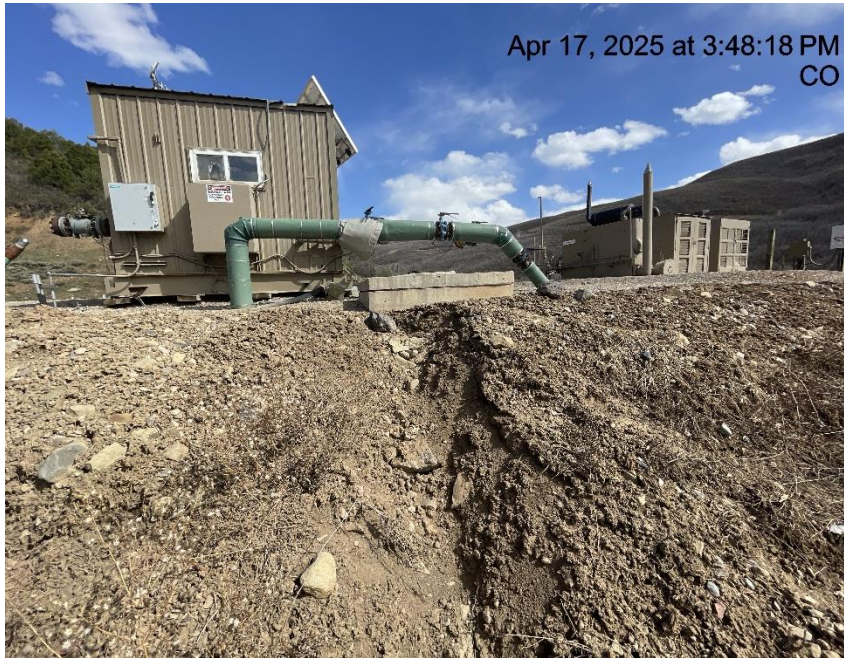
Photo # 2905 Erosion & transport of sediment off location /berm needs maintenance
