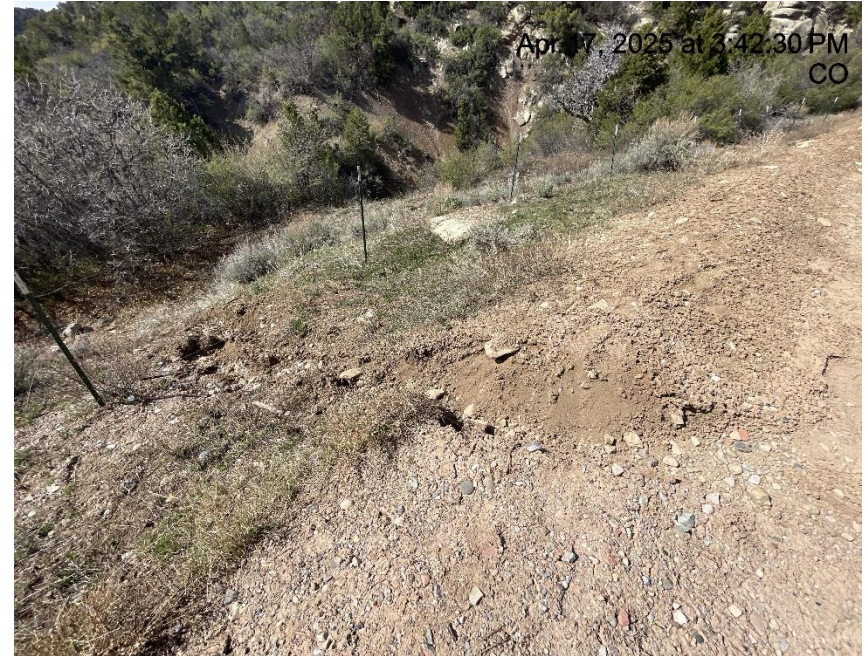
Photo # 2893 Erosion & transport of sediment off location /berm needs maintenance
