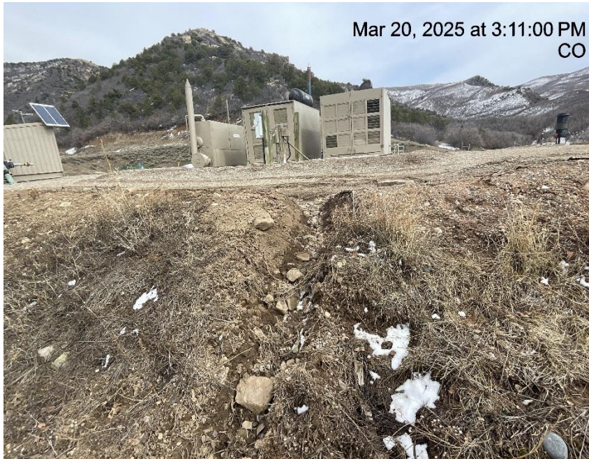
Photo # 6261 From inspection 708906071 conducted on 03/20/2025 Erosion & transport of sediment off location /berm needs maintenance
