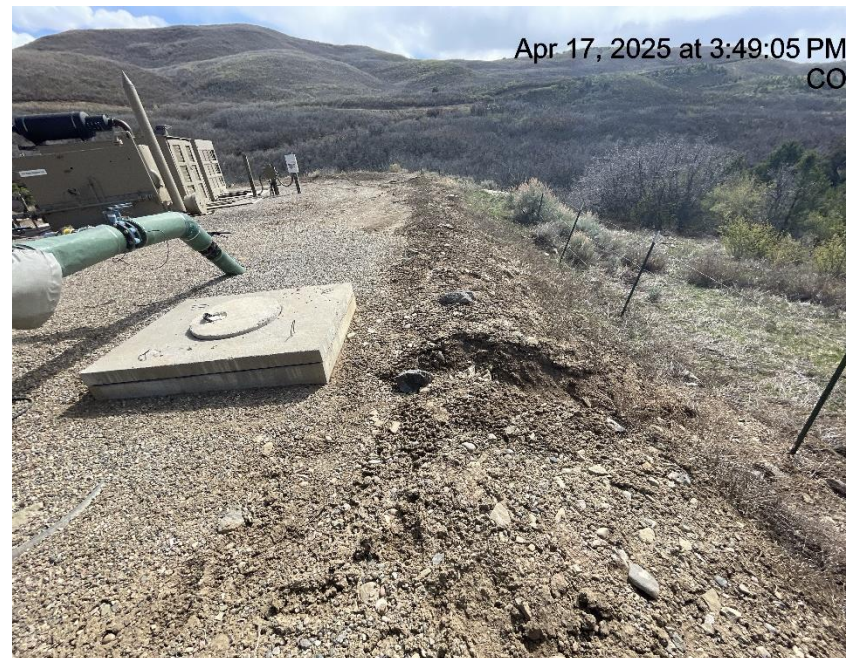
Photo # 2902 Erosion & transport of sediment off location /berm needs maintenance
