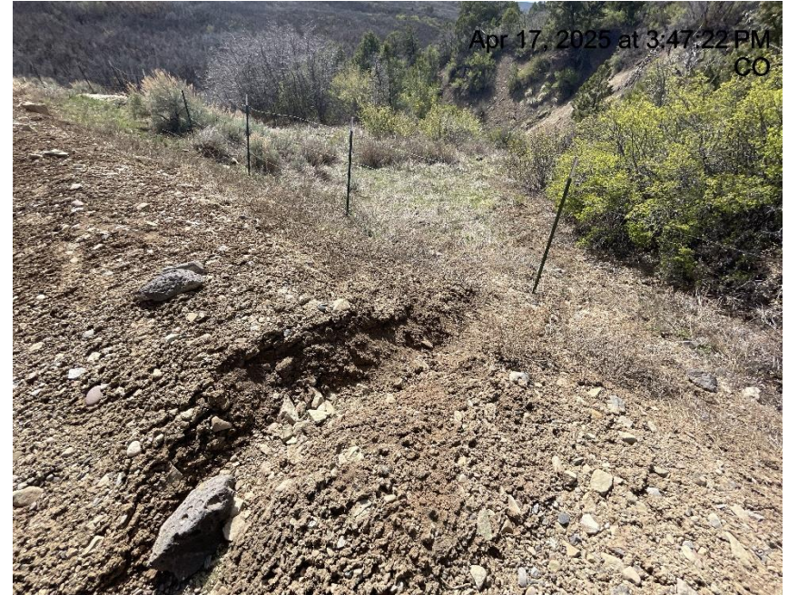
Photo # 2904 Erosion & transport of sediment off location /berm needs maintenance
