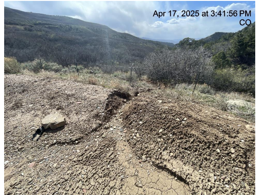
Photo # 2892 Erosion & transport of sediment off location /berm needs maintenance
