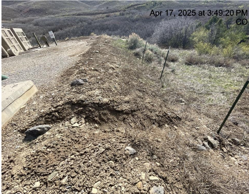
Photo # 2903 Erosion & transport of sediment off location /berm needs maintenance
