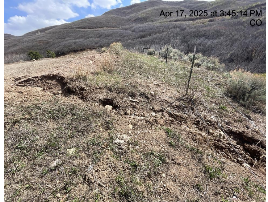
Photo # 2896 Erosion & transport of sediment off location /berm needs maintenance
