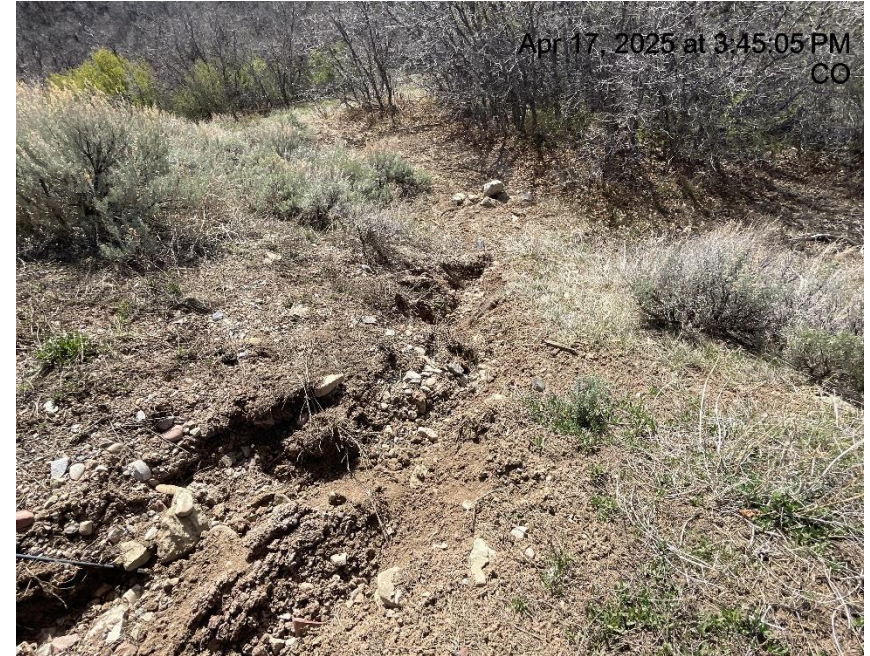
Photo # 2898 Erosion & transport of sediment off location /berm needs maintenance
