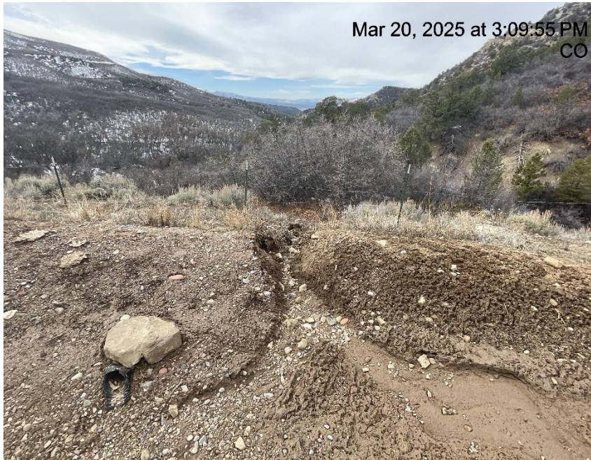
Photo # 6258 From inspection 708906071 conducted on 03/20/2025 Erosion & transport of sediment off location /berm needs maintenance
