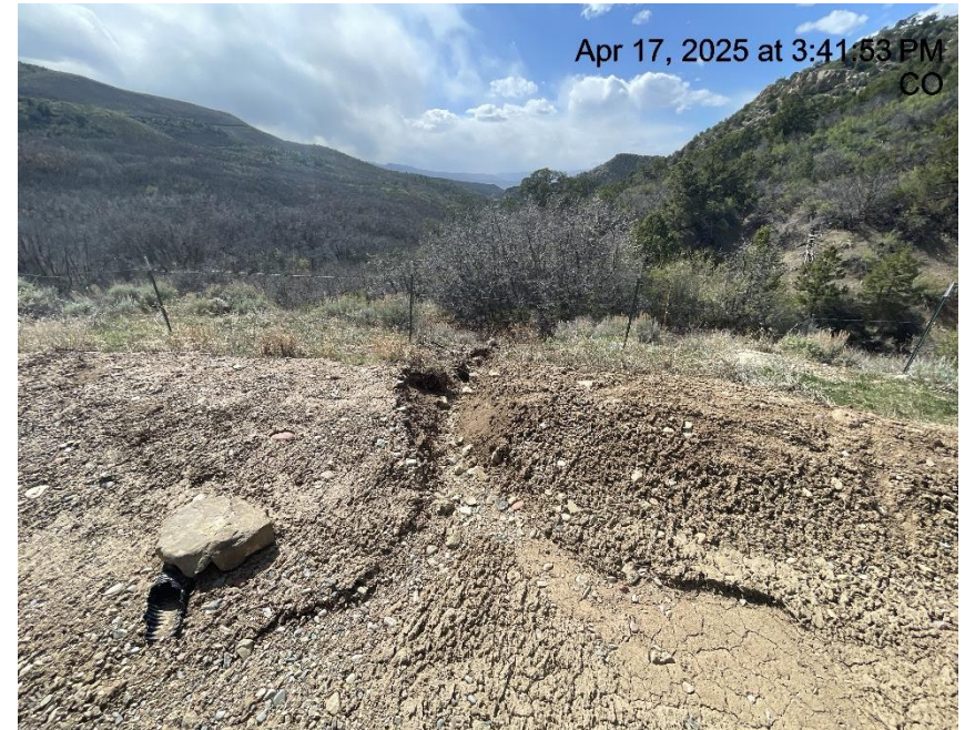
Photo # 2891 Erosion & transport of sediment off location /berm needs maintenance
