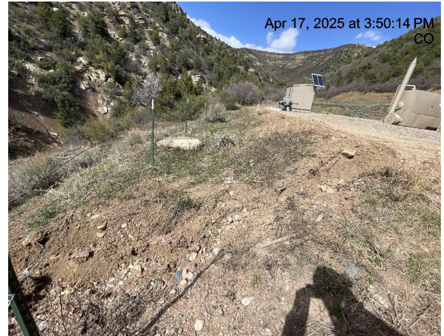
Photo # 2900 Erosion & transport of sediment off location /berm needs maintenance
