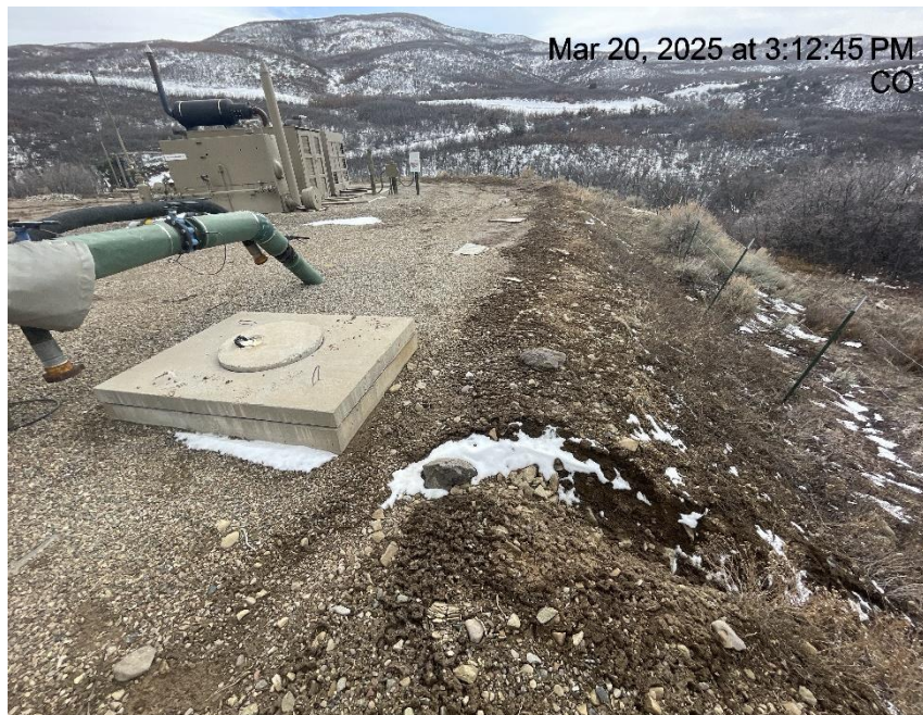
Photo # 6263 From inspection 708906071 conducted on 03/20/2025 Erosion & transport of sediment off location /berm needs maintenance
