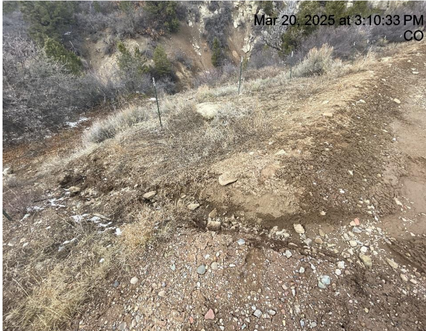
Photo # 6260 From inspection 708906071 conducted on 03/20/2025 Erosion & transport of sediment off location /berm needs maintenance
