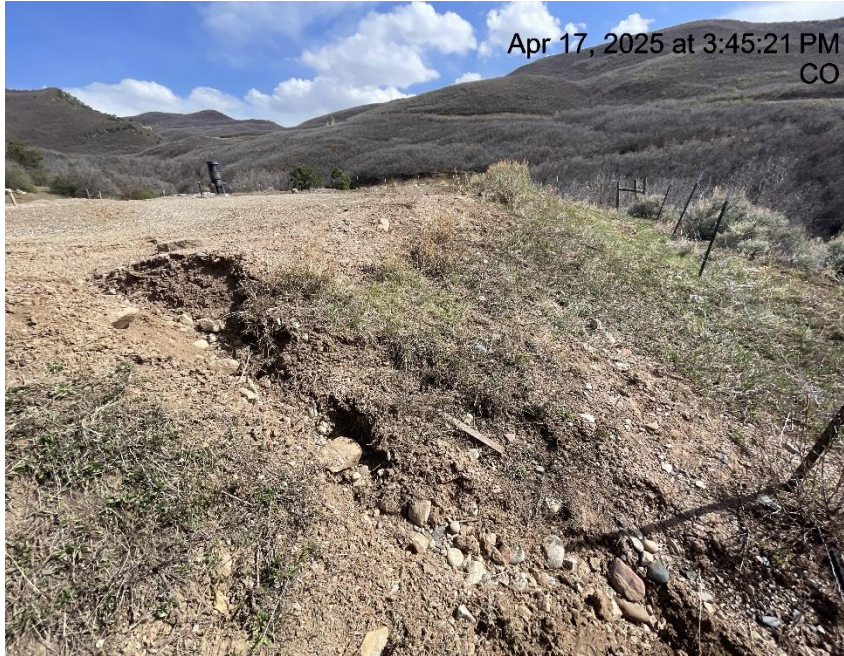
Photo # 2895 Erosion & transport of sediment off location /berm needs maintenance
