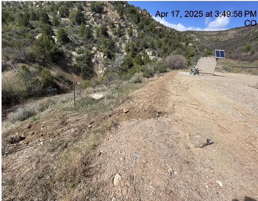
Photo # 2899 Erosion & transport of sediment off location /berm needs maintenance
