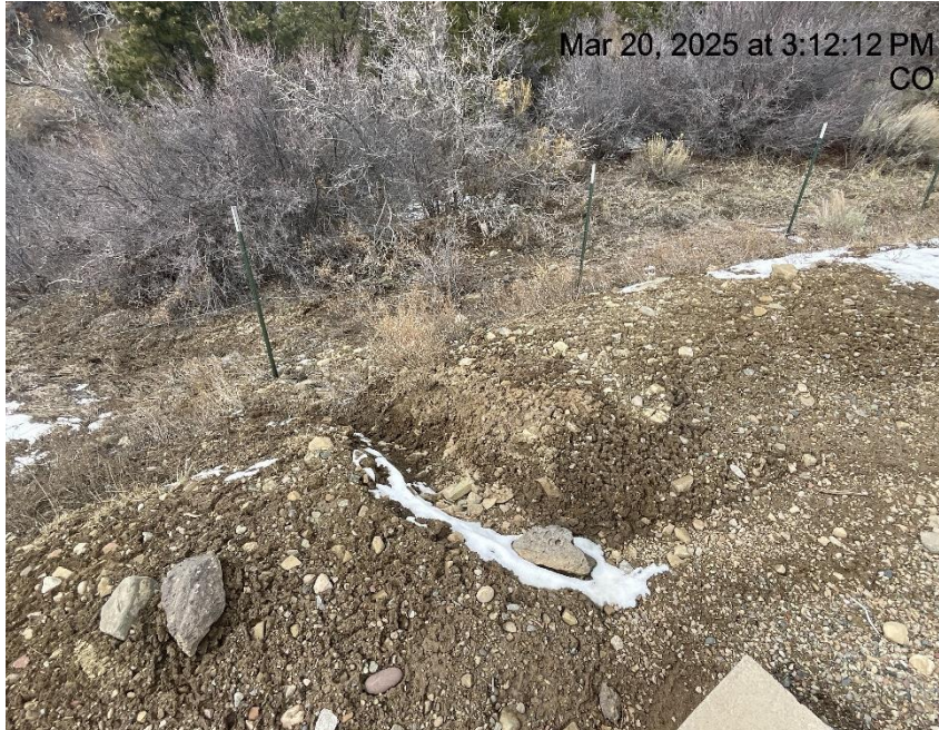
Photo # 6262 From inspection 708906071 conducted on 03/20/2025 Erosion & transport of sediment off location /berm needs maintenance
