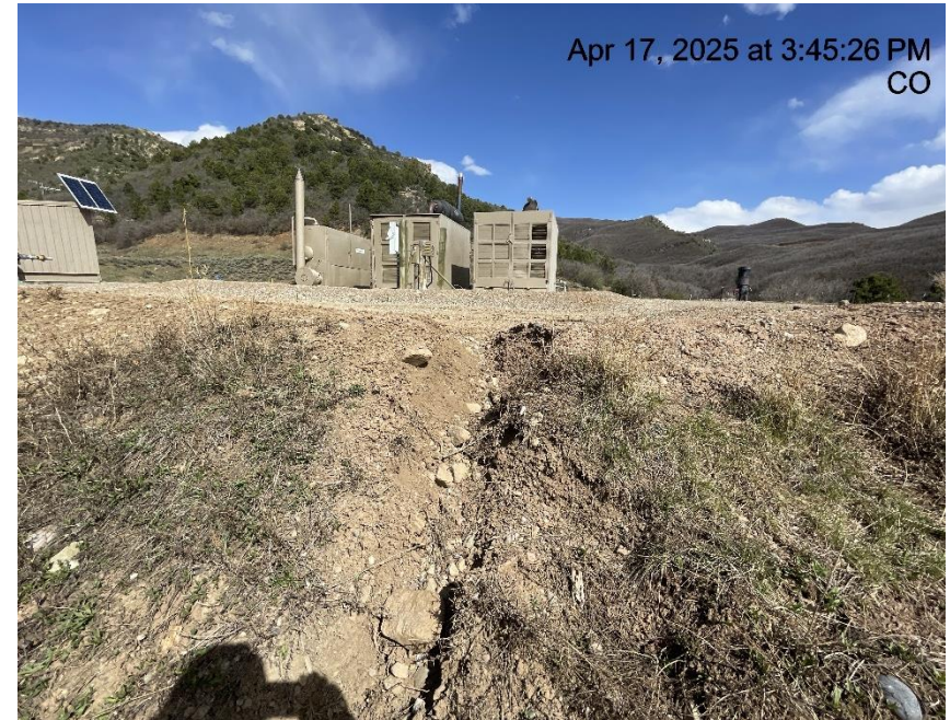
Photo # 2894 Erosion & transport of sediment off location /berm needs maintenance
