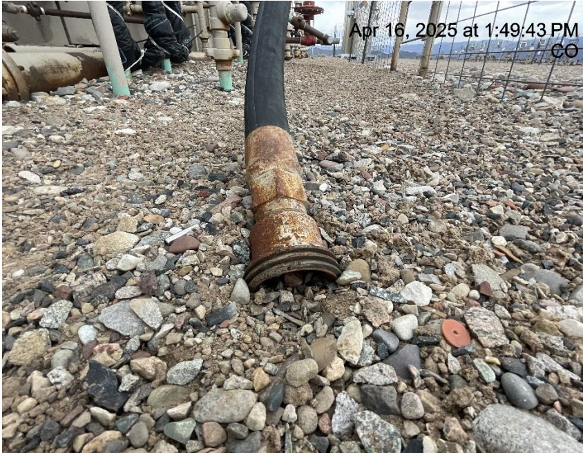
Photo # 2066 Open ended kelly hose/wildlife hazard /available for entry by wildlife
